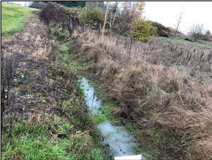
Photograph 5: Standing water observed in drainage ditch at the south parcel boundary of parcel no. 214247000, running east-west.
