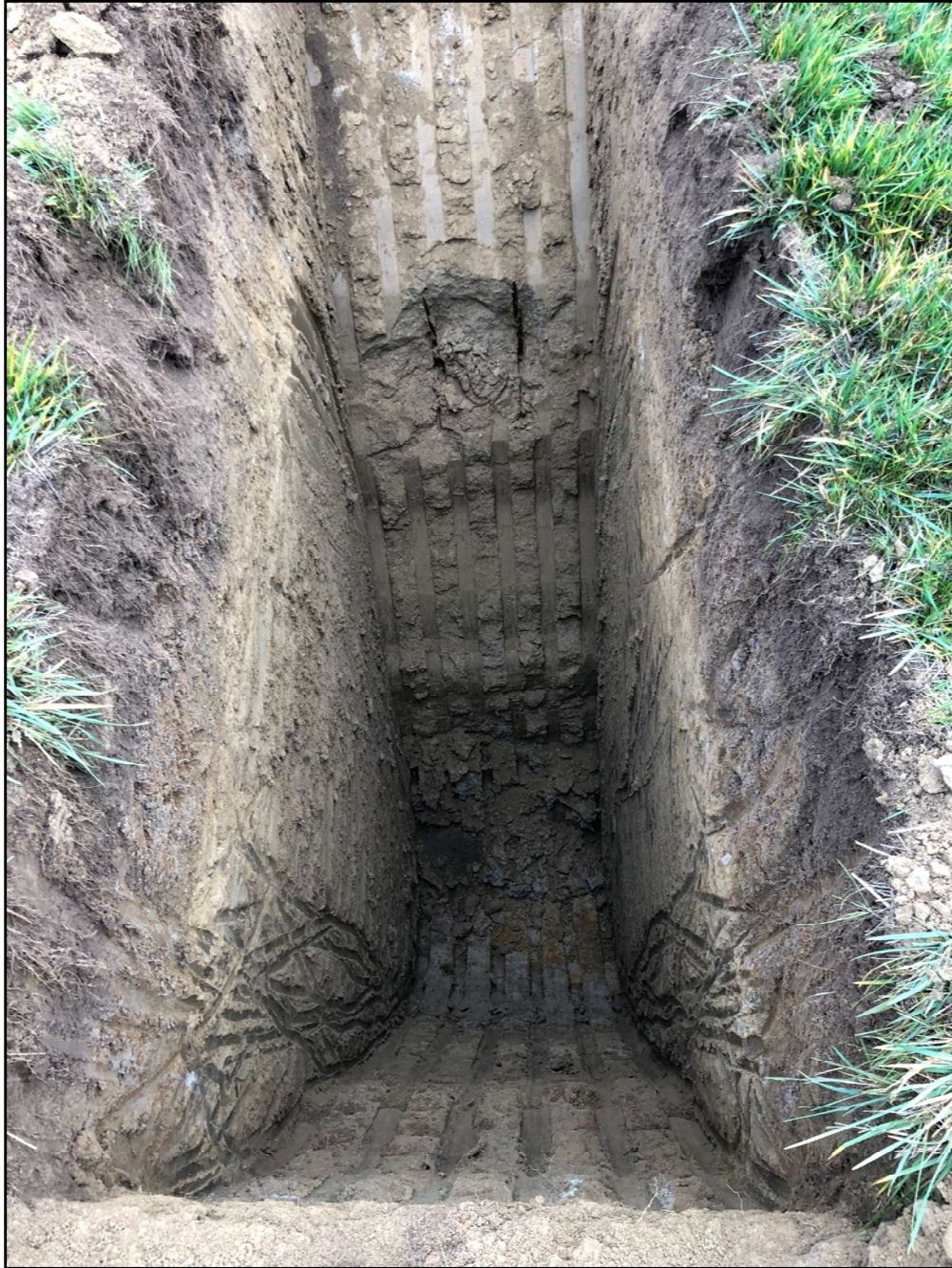
Test Pit TP-4
