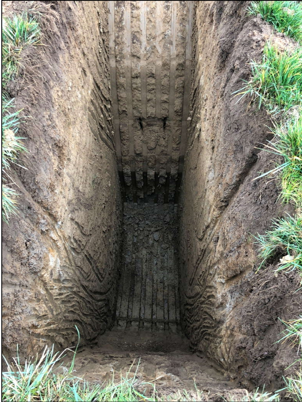
Test Pit TP-3
