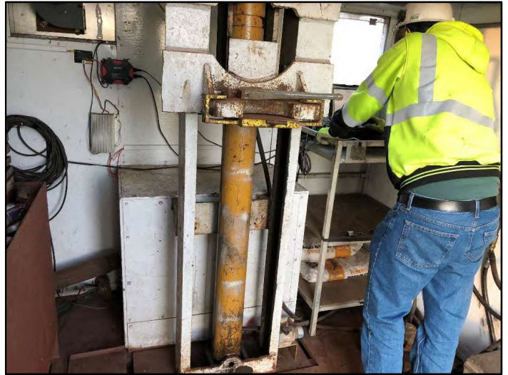
Photograph 2: Inside of track-mounted CPT apparatus, running porewater dissipation testing for CPT-1.
