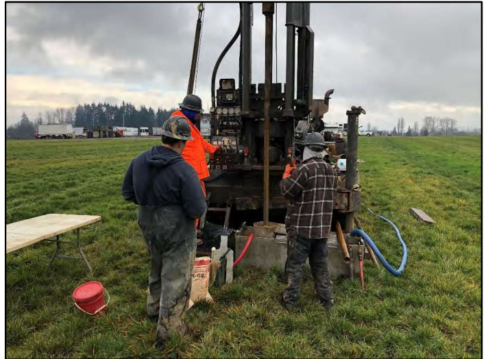
Photograph 8: Site exploration activity with mud-rotary drill apparatus, soil boring SB-1.
