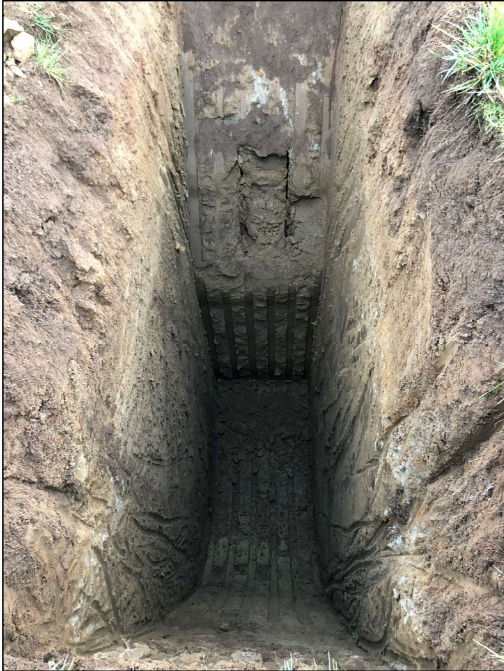
Test Pit TP-1
