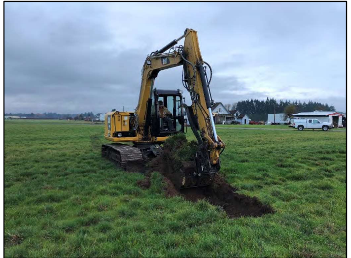
Photograph 4: Site exploration observations, test pit TP-1.
