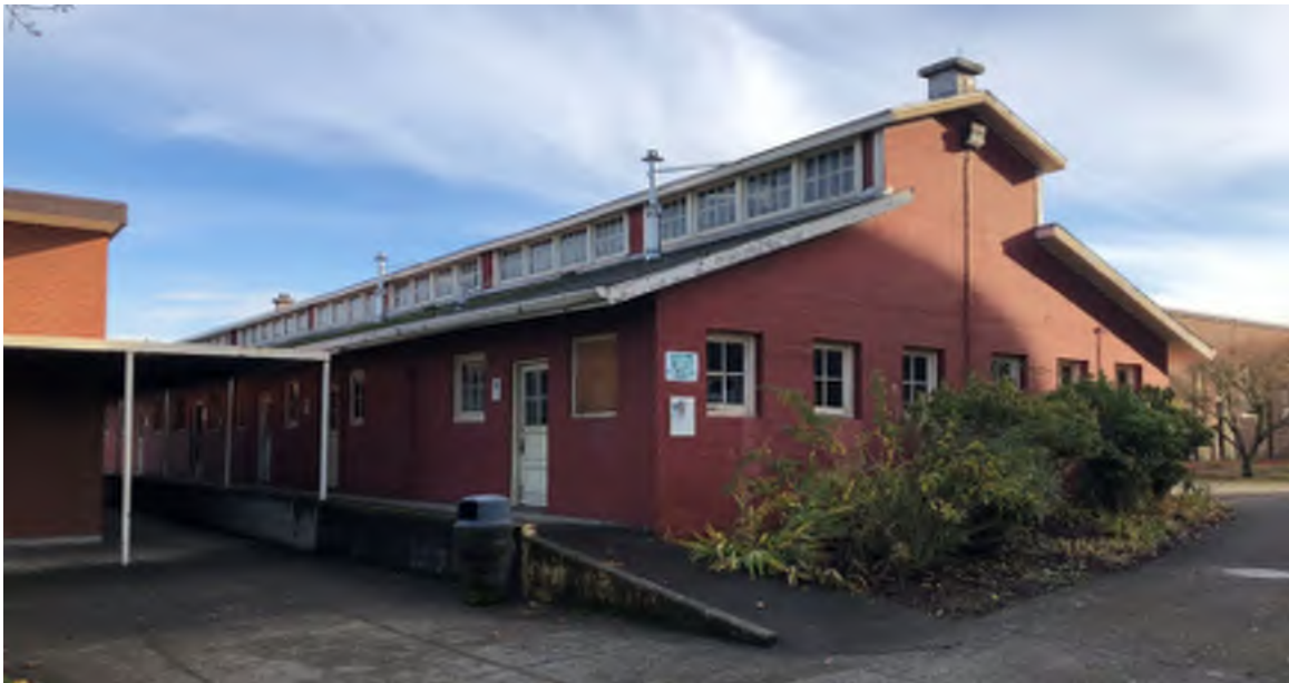
Maintenance/Storage from the Northwest
