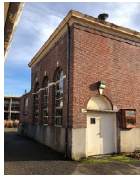
Boiler House from Northeast
