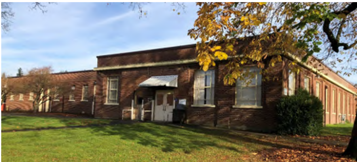
Kitchen/Cafeteria from the southeast
