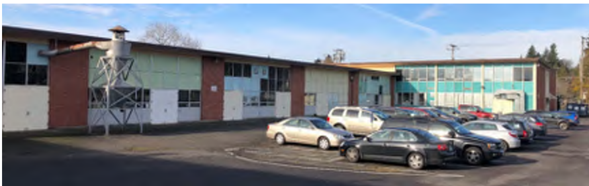
Epperson from the Southeast (1-story Shop Wing)
