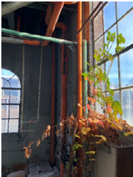
Boiler House interior with plant growth
