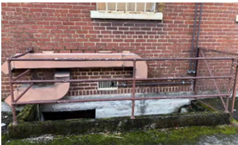
Exterior stair to utility tunnel under building
