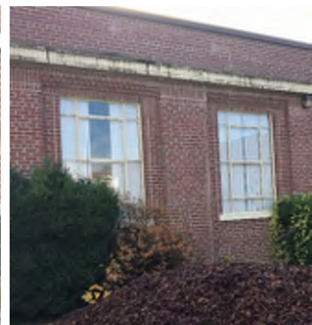
Exterior wall at Dining Room addition.
