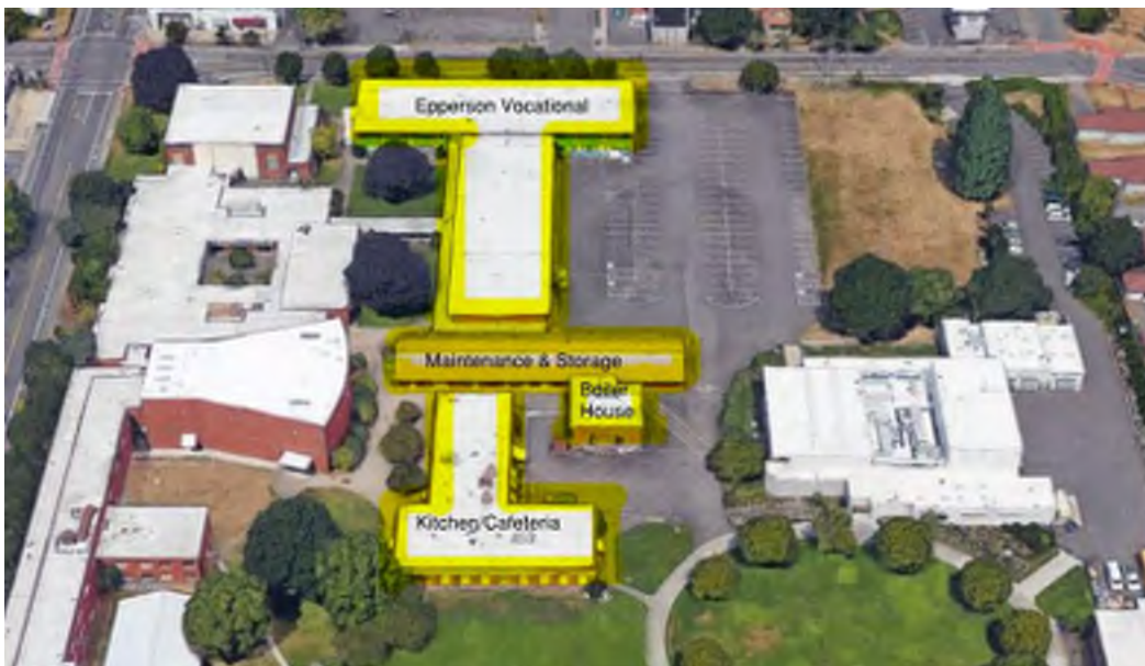
Aerial of CCDHL Campus with buildings to be demolished highlighted
