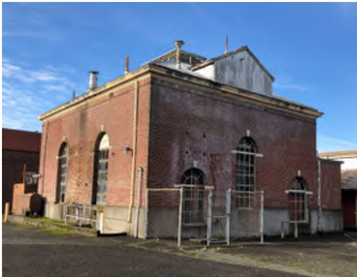
Boiler House from Southwest
