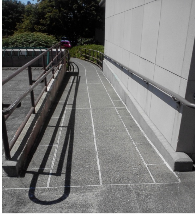
Photo 10. Concrete Ramp (Top)
