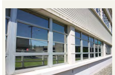
Windows and etched concrete exterior
