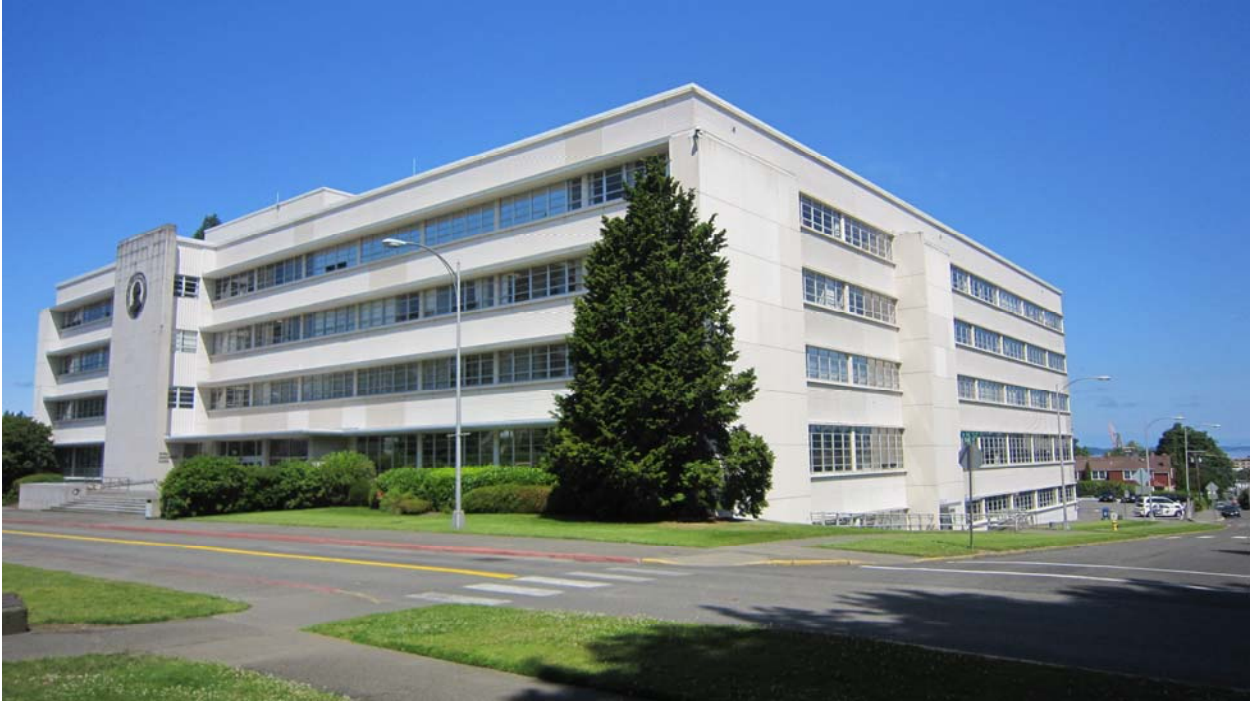
GA Building East and South Side
