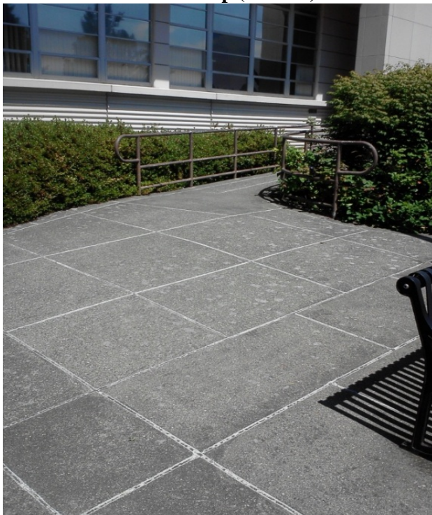
Photo 11. Concrete Ramp (Bottom)
