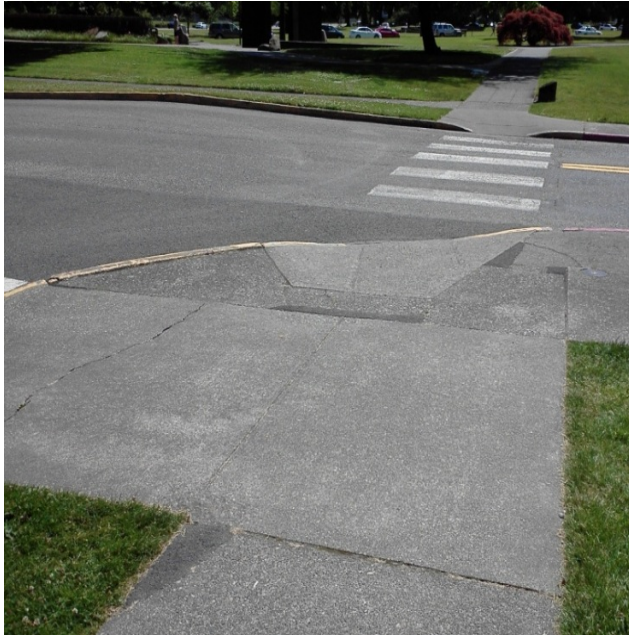
Photo 1. Cracked Sidewalk
