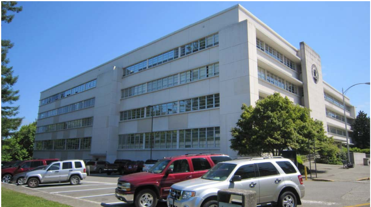
GA Building West Side
