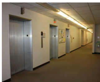
Third floor elevator lobby
