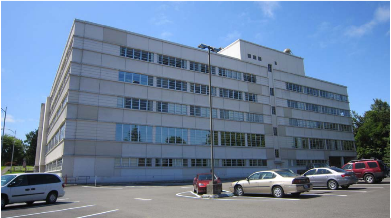
GA Building North Side
