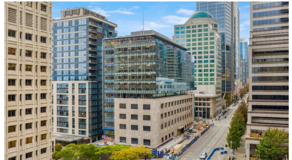
Federal Reserve Building, Seattle, Washington
