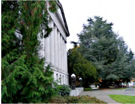
Trees & tall shrubs crowd walls. Beyond: heritage cedar suffers from compaction & drops limbs in storms.
