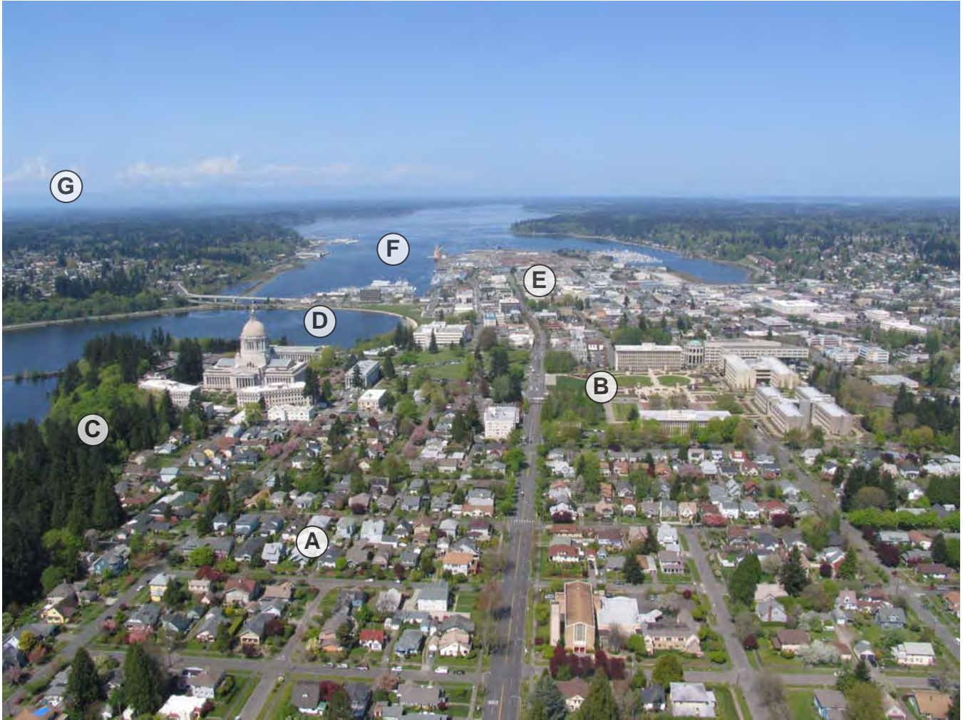
Fig. 3.6 Aerial View looking north showing the Capitol and many of the essential components of the surrounding context: A) The South Capitol Neighborhood (National Register Historic District), B) the East Campus, C) the Native Forest edge, D) Capitol Lake, E) Olympia, F) Budd Inlet, G) the Olympic Mountains (2006, Photo Source: Washington State Department of Transportation)
