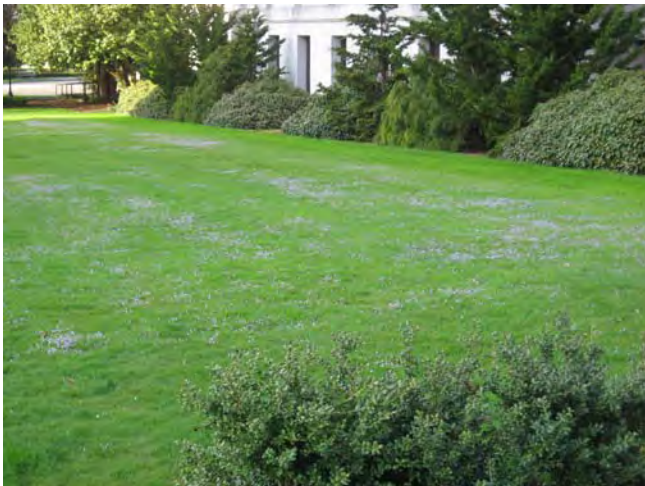
Fig. 10.1.6 Veronica in lawn indicates poor drainage. Shrubs beyond obscure windows and crowd building (April 2009, Source: Arbutus Design)
