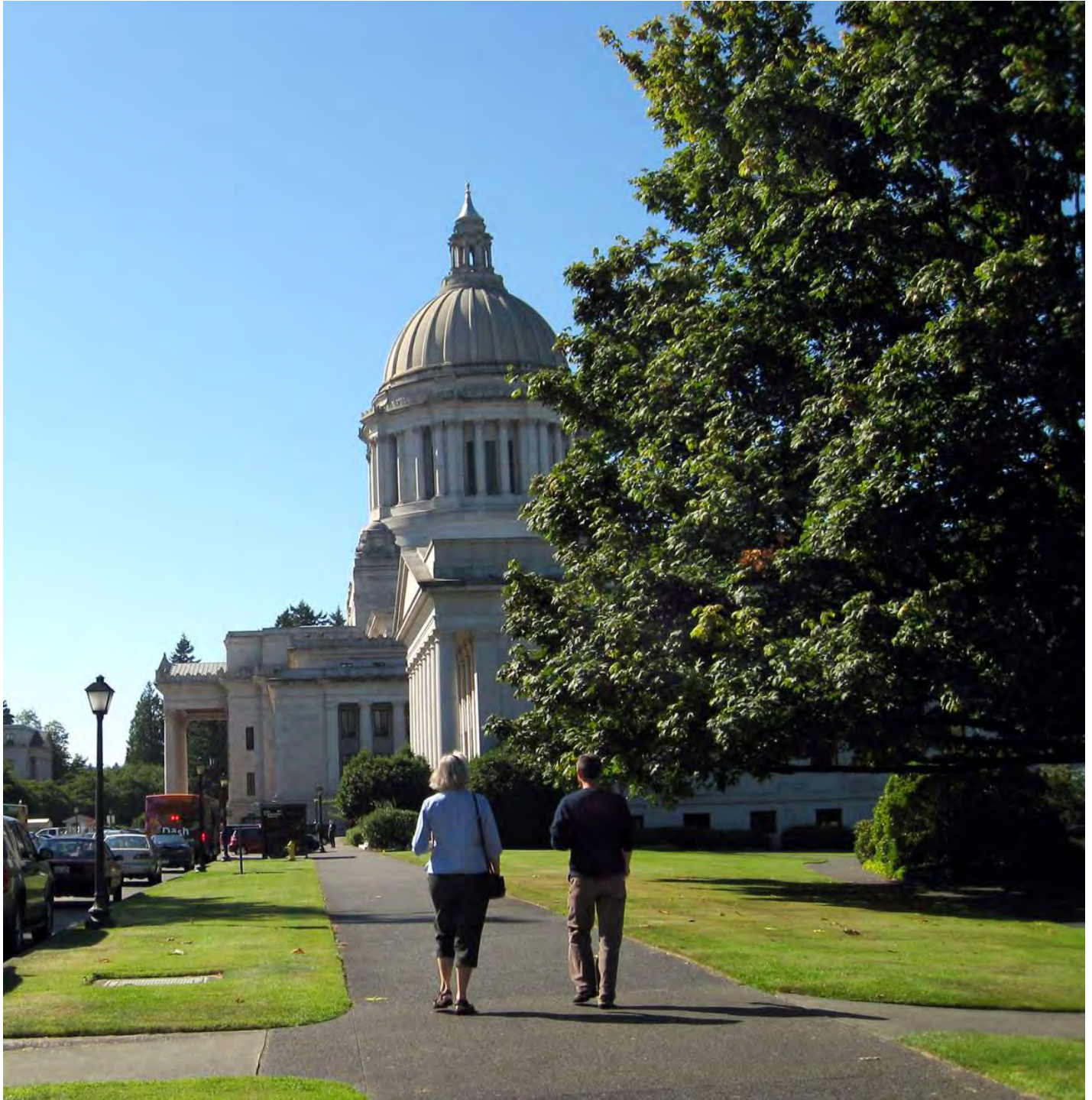
Fig. 4.2 Pedestrian approach to Capitol Group along Sid Snyder Avenue (Sept. 2008, Source: Mithun)
