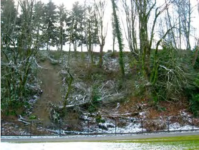
Fig. 10.3.28 Tree uprooted by recent north bluff landslide further opens canopy to invasives and soil to erosion. (March 2009, Source: Arbutus Design)
