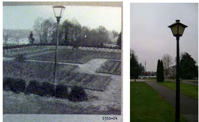
Figure 11.6 Comparison of historic and current carriage lantern lighting poles [source: Frederick Law Olmsted National Historic Site, National Park Service (historic photo), Dark|Light Consulting, LLC (2009 photo)]
