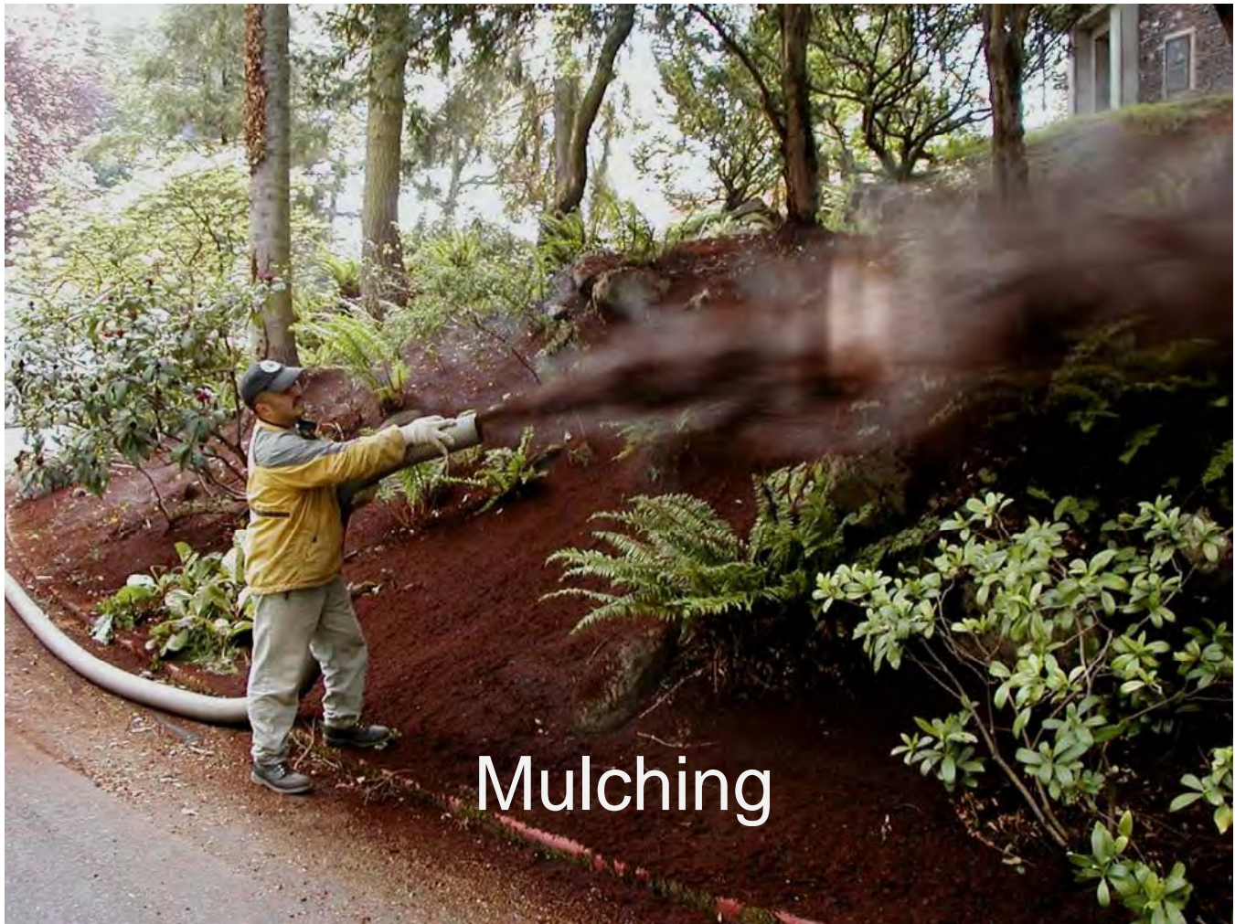
Fig. 10.5.2 Organic mulches improve soil health & fertility and reduces compaction. (2004, Source: Seattle Parks and Recreation)
