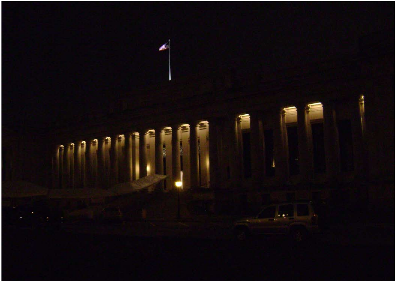
Figure 11.1 Lighting at porticos of Temple of Justice (source:Dark|Light Consulting, LLC, 2009)
