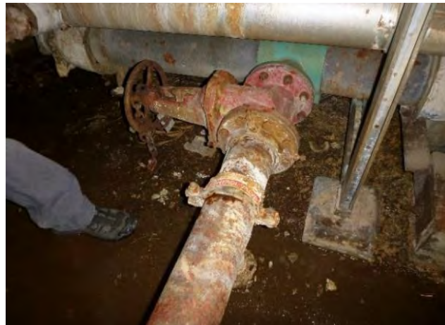
Figure 2. Aged Steam Distribution System
