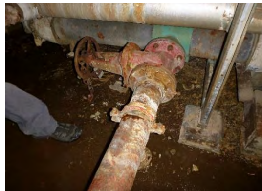
Figure 6. Aged Steam Distribution System
