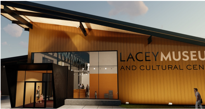
City of Lacey, Museum and Civic Center, Targeted LEED Silver
