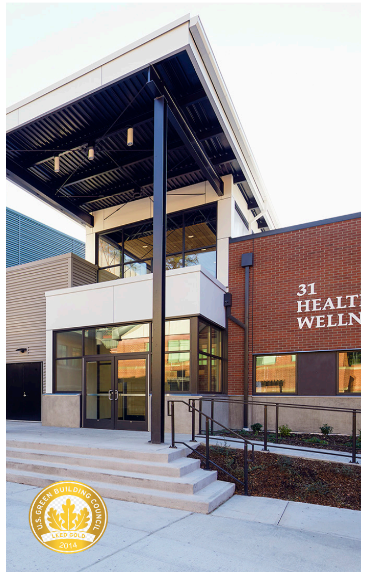
South Puget Sound Community College Health And Wellness, LEED Gold
