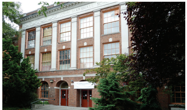
SPS JOHN MARSHALL SCHOOL | CONDITION ASSESSMENTS
