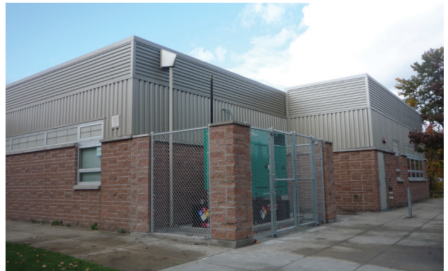
EDMONDS SD MEADOWDALE HS | GENERATOR REPLACEMENT
