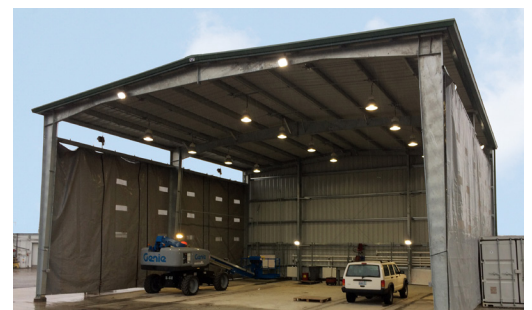
KCSW CAT SHACK REPLACEMENT
