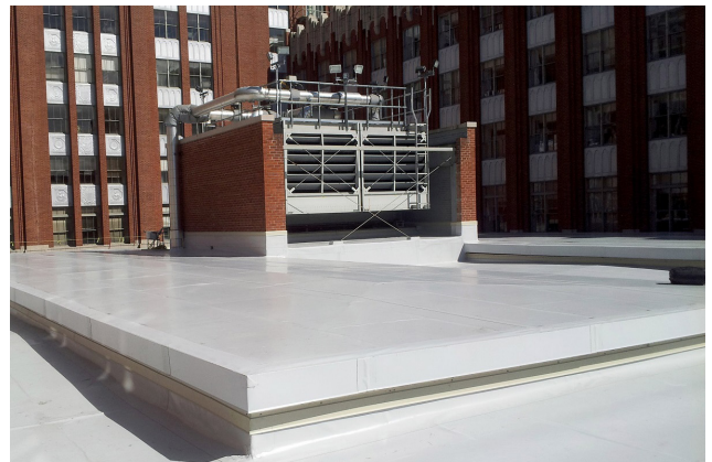
US GSA FEDERAL OFFICE BUILDING | ROOF REPLACEMENT
