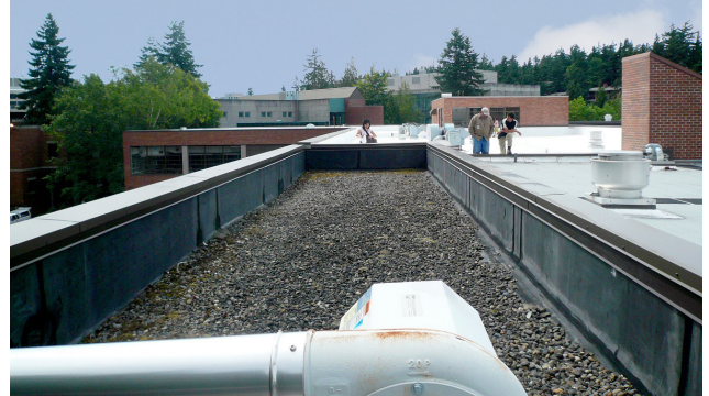
WWU FINE ARTS BUILDING | ROOF REPLACEMENT
