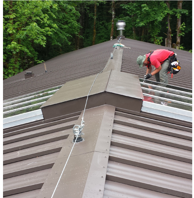
TESC LONG HOUSE | ROOF ASSESSMENTS
