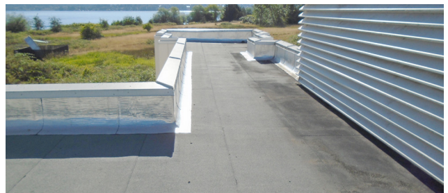
NOAA WRC | ROOF ASSESSMENT
