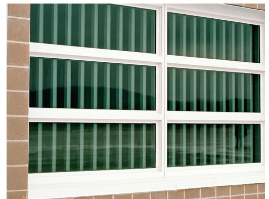
CORRECTIONAL FACILITY | WINDOW REPLACEMENTS
