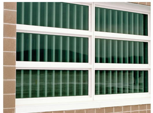
CORRECTIONAL FACILITY | WINDOW REPLACEMENTS
