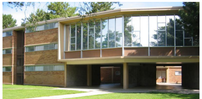
CWU STEPHENS-WHITNEY HALL | TENANT IMPROVEMENTS
