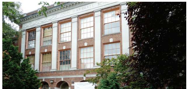
SPS JOHN MARSHALL SCHOOL | CONDITION ASSESSMENTS
