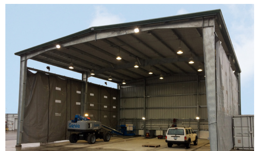
KCSW CAT SHACK REPLACEMENT
