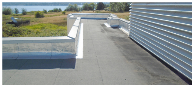
NOAA WRC | ROOF ASSESSMENT
