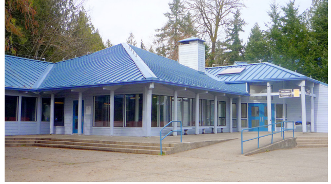
TESC HCC BUILDING | ROOF REPLACEMENT
