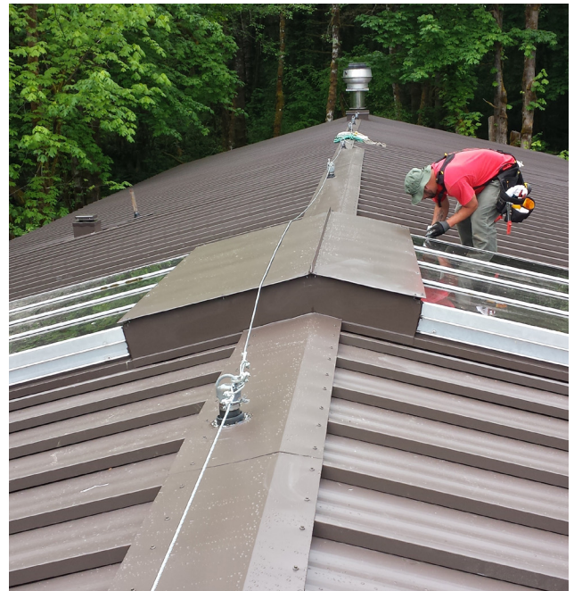
TESC LONG HOUSE | ROOF ASSESSMENTS
