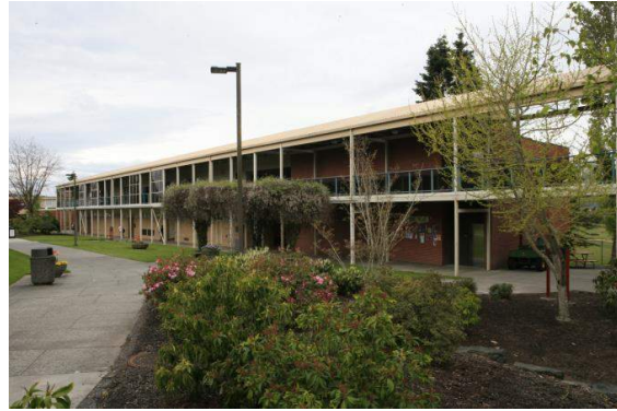
South facade, partial 2014
