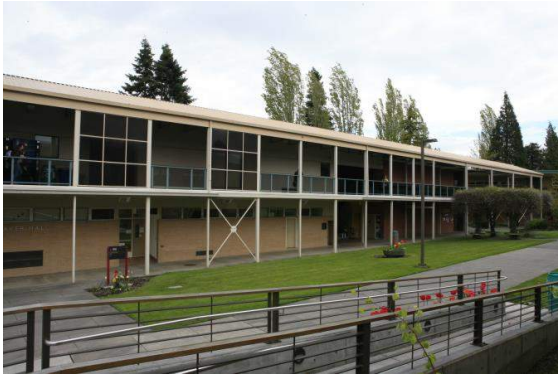
South facade, partial 2014
