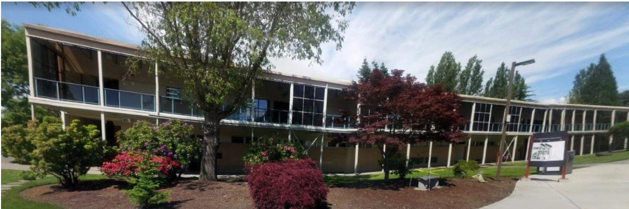
Photo 2. Google Maps view of front of building
