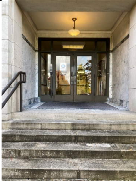
North Entry doors, sandstone steps
