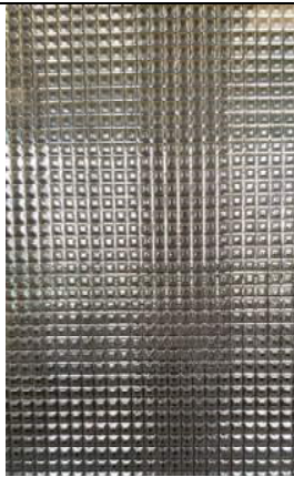
Glass detail in door panel
