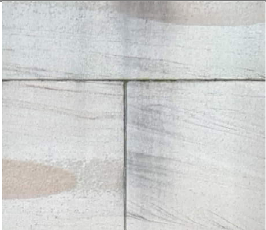
Wilkeson Sandstone smooth panels at building base
