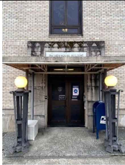
South Entry doors, sandstone surround, variegated glazed brick, lamps (quantity: 2)
