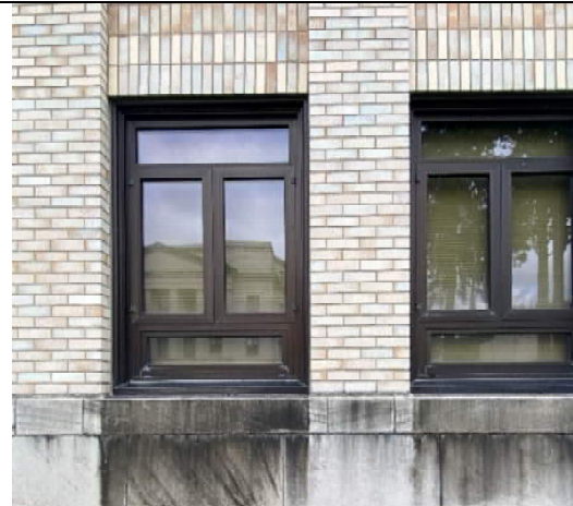
Aluminum Windows and Wilkeson Sandstone sills
