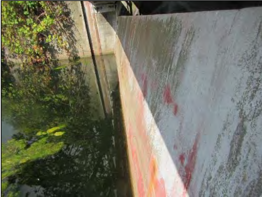
Photograph 18: Lake Site of West Radial Gate.
