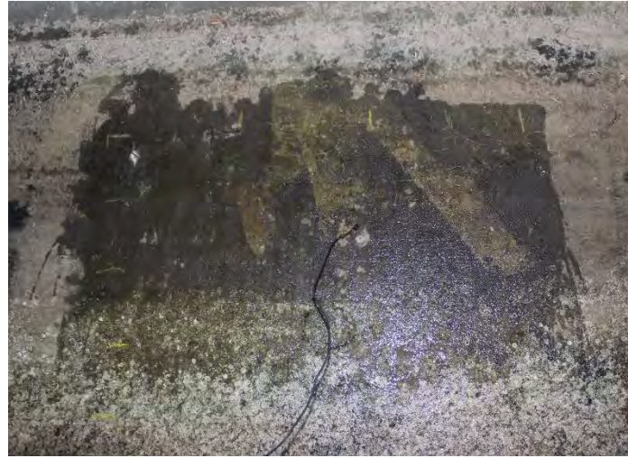
Figure 23: Half-Cell Potential Survey Site (West Channel Pier Wall – High Tidal Zone)
