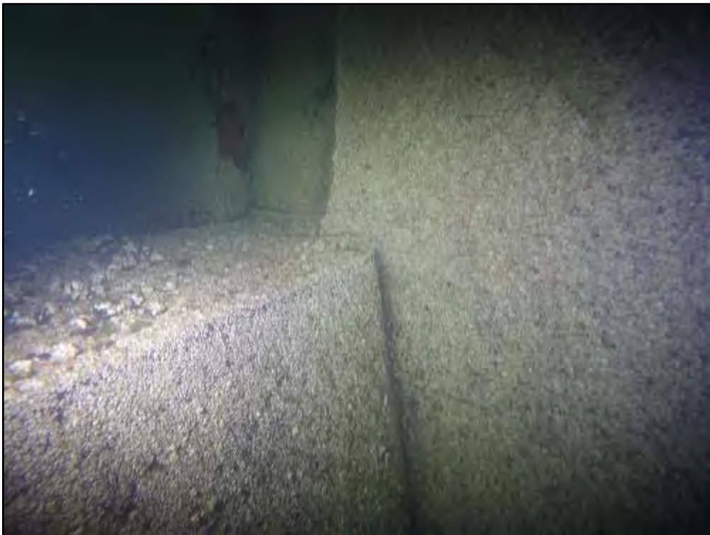
Photograph 45: Interface of Sill, Stoplog Cutout, and Pier Wall Underwater
