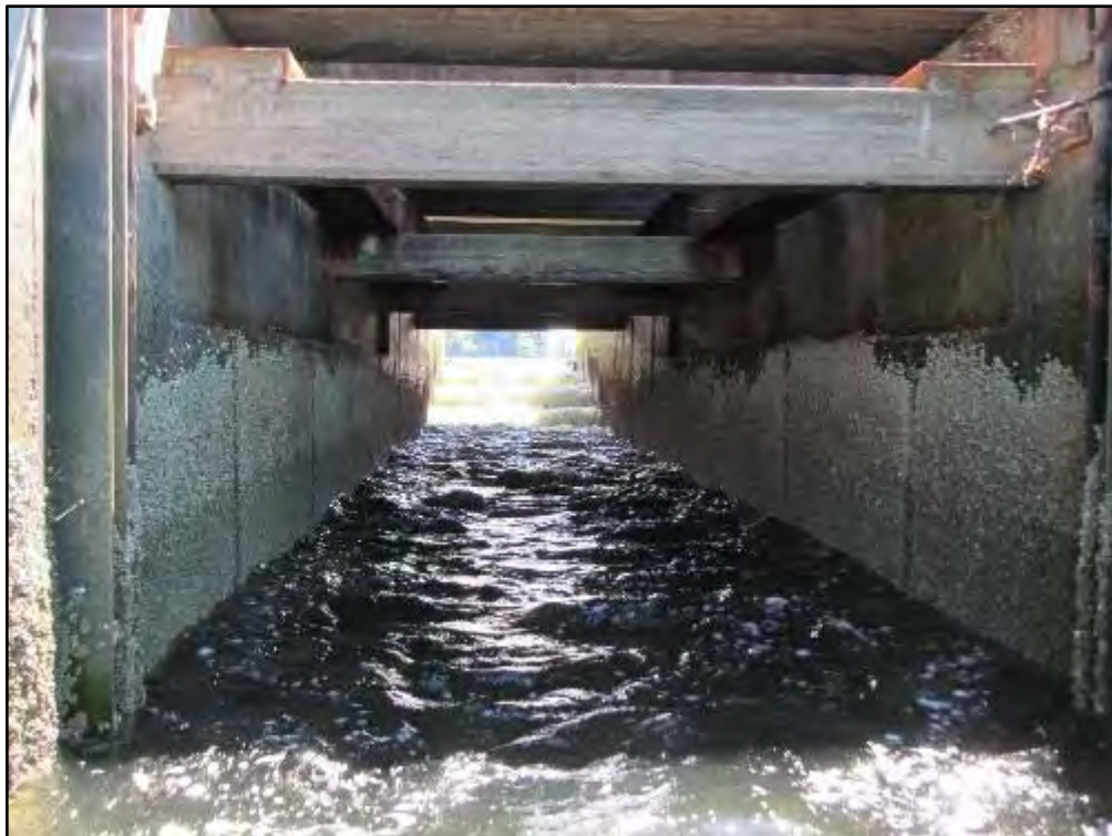
Photograph 3: Typical Pier Wall at Fish ladder
