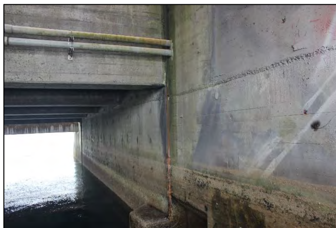
Figure 3: West Channel Pier Wall
