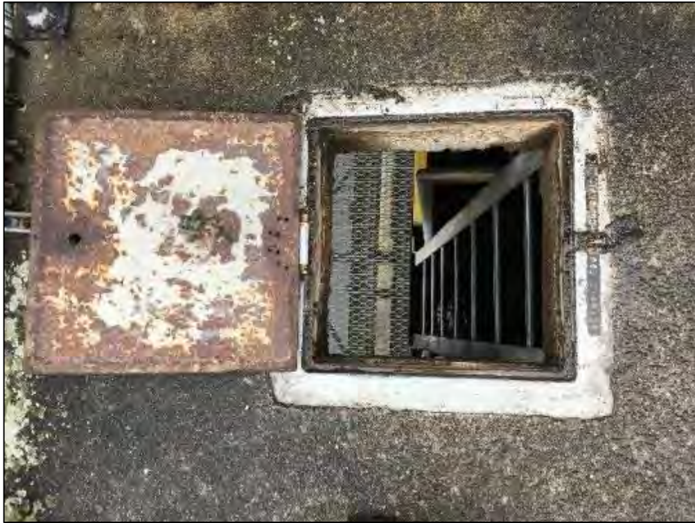
Photograph 33: Catwalk Access Ladder Opening
