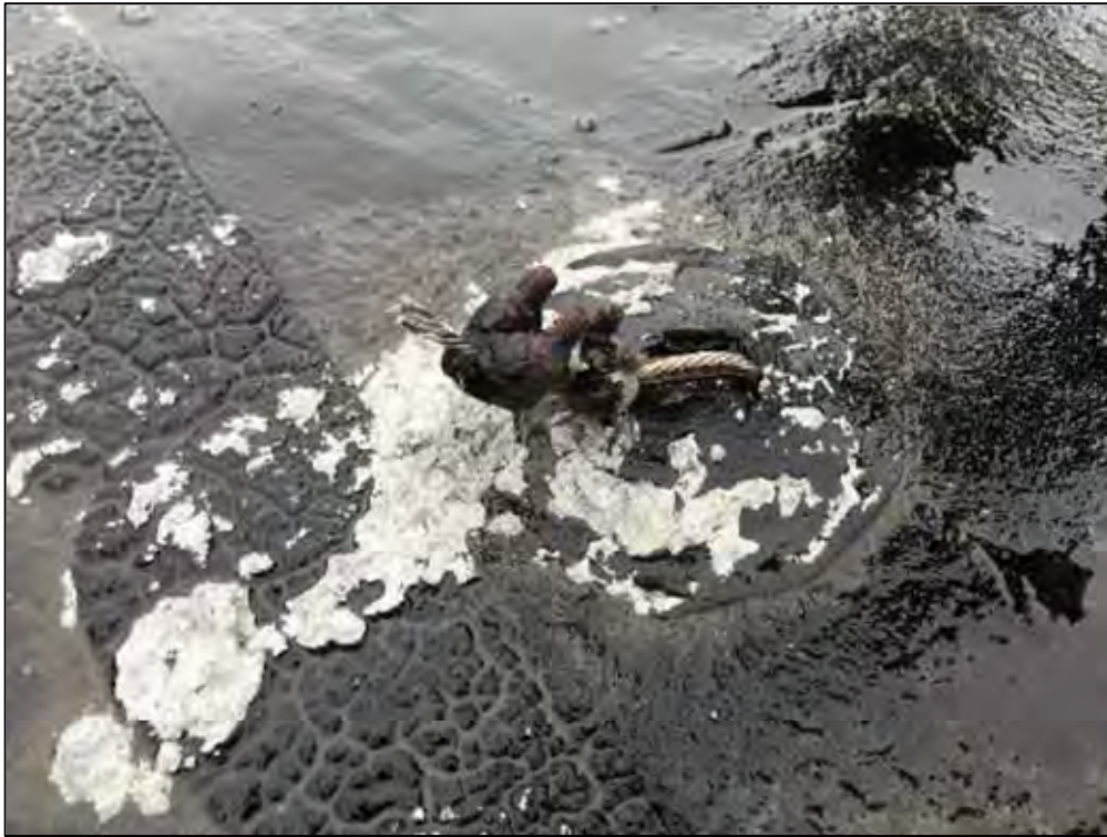
Photograph 39: Alligator Cracking of the Control Room's Roof Membrane and a Failed Fall-Protection Anchor Point
