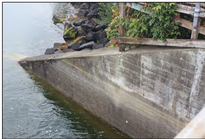
Figure 2: East Wing Wall – Budd Inlet Side
