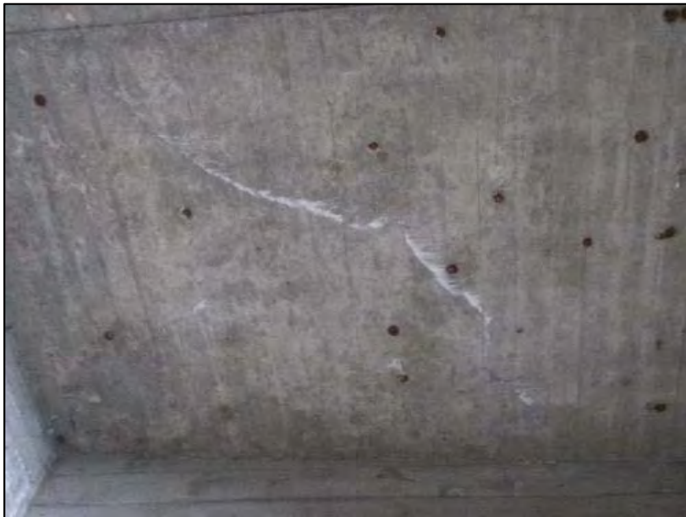
Photograph 16: Typical Deck Soffit – West Channel
