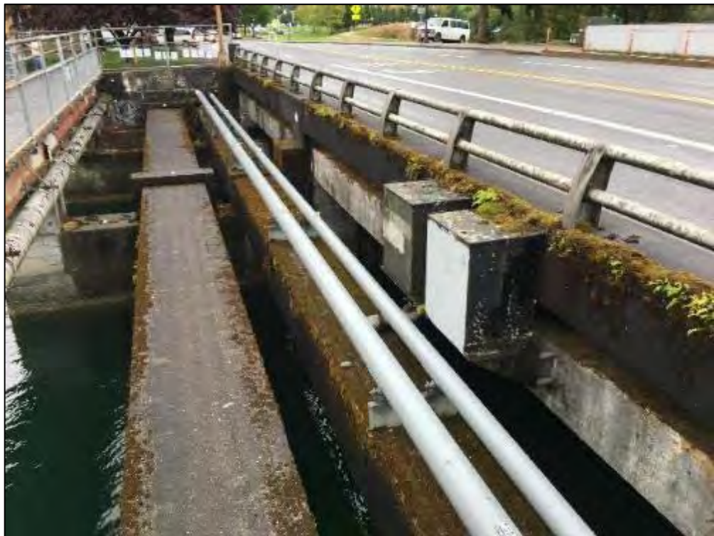
Photograph 29: Typical Condition of the Utilities Crossing the Dam
