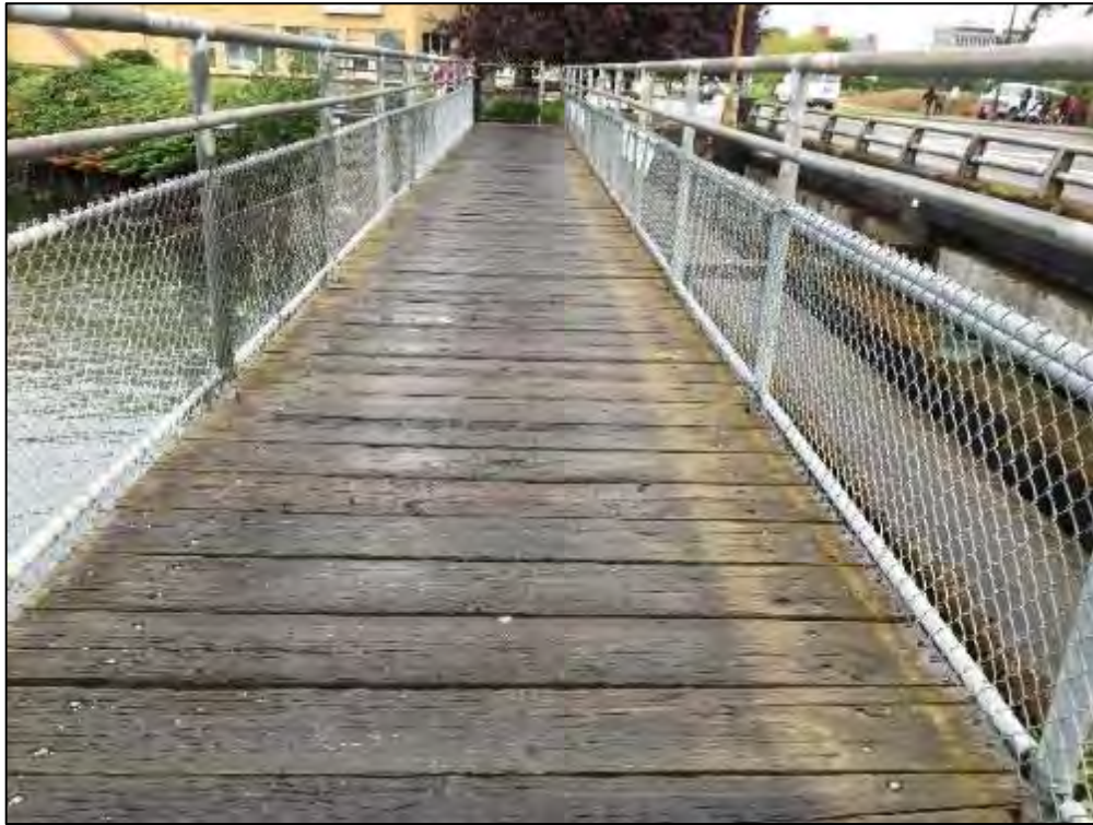
Photograph 25: Topside of the Walkway, Looking East
