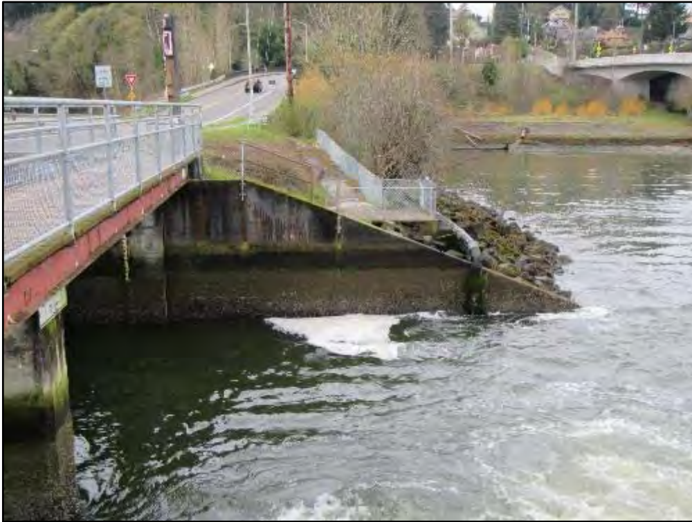
Photograph 42: West Downstream Wingwall
