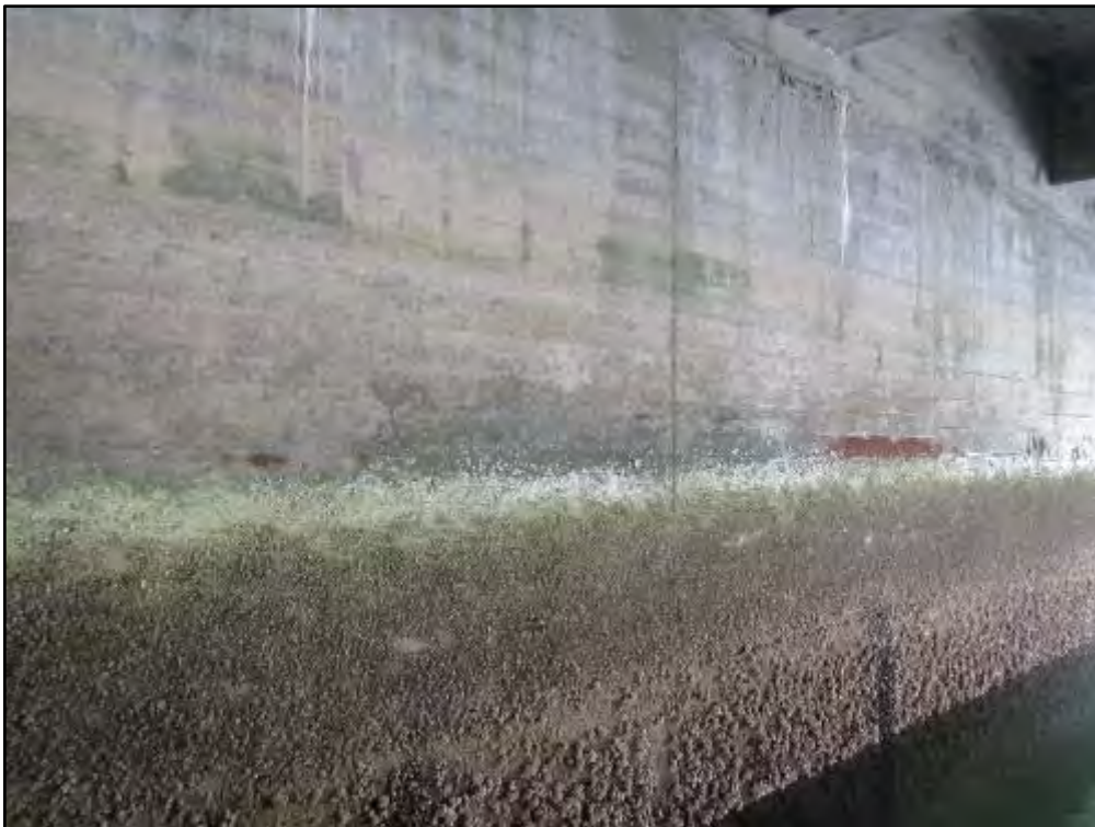
Photograph 43: Typical Abutment Looking Northwest
