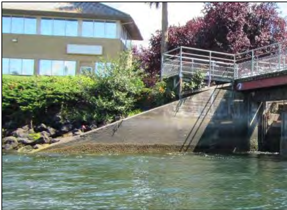
Photograph 1: East Downstream Wingwall
