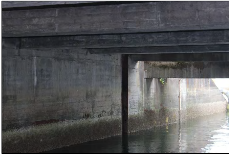
Figure 4: West Channel Abutment Wall
