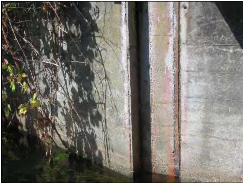
Photograph 47: Stoplog Cutout on West Upstream Abutment
