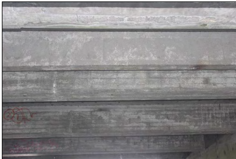
Figure 5: East Channel Deck Soffit and Girders
