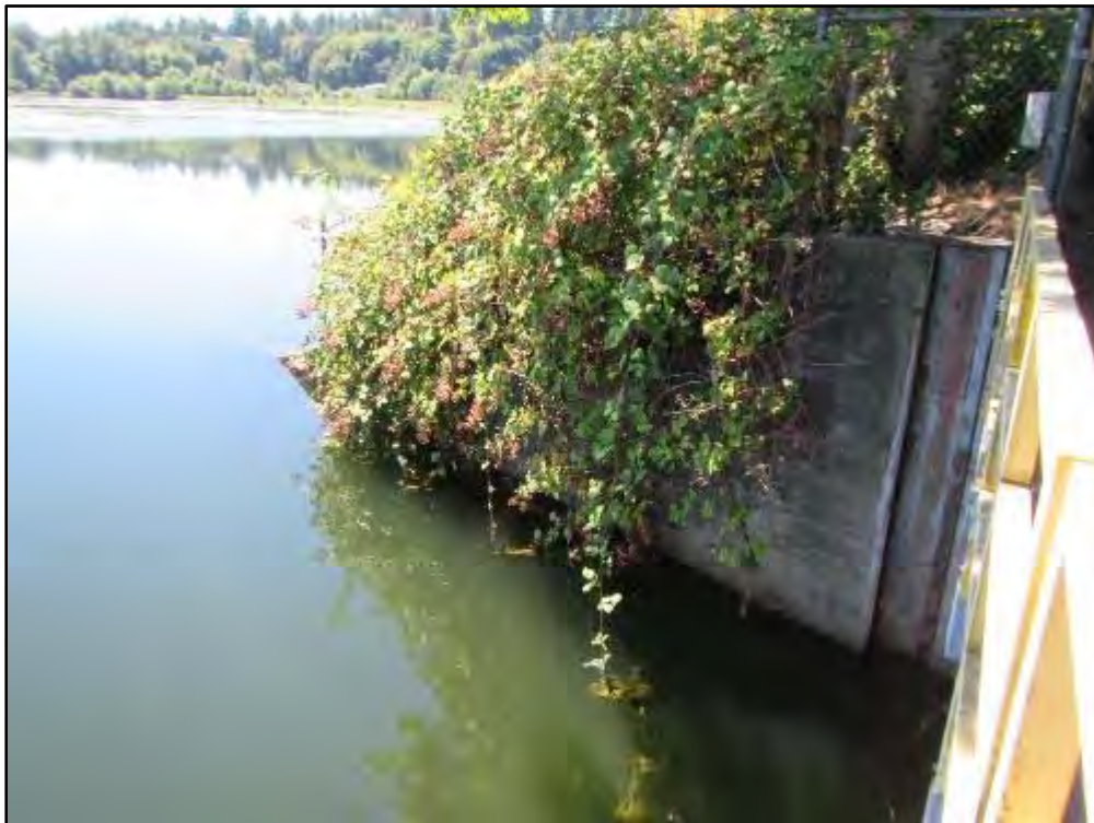
Photograph 41: West Upstream Wingwall
