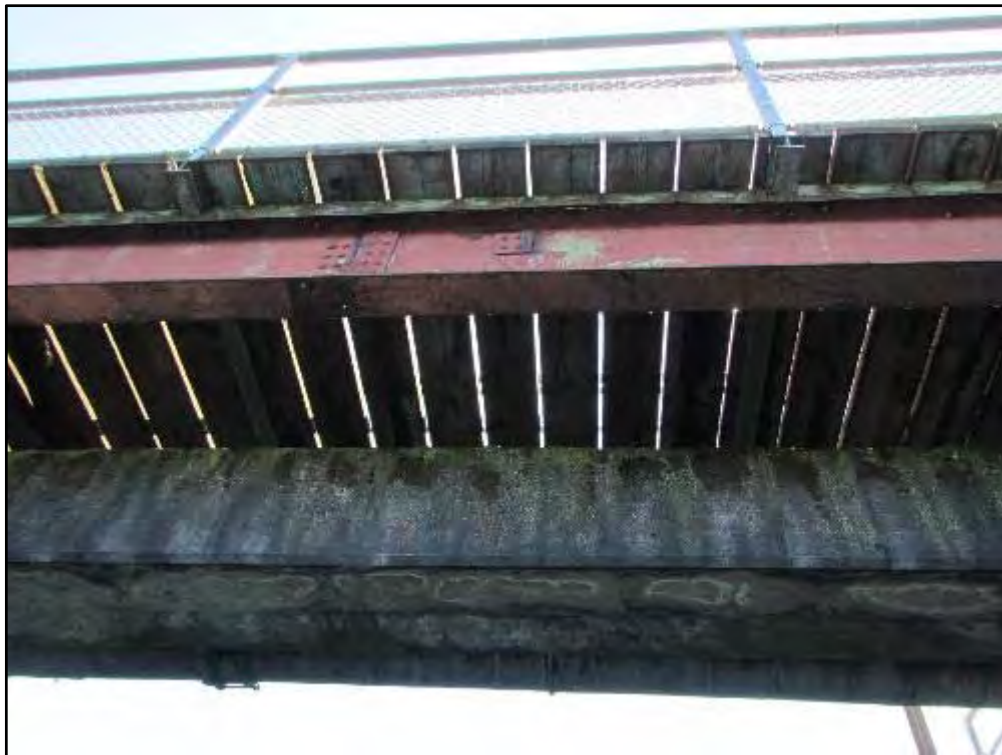
Photograph 24: Underside of the Walkway
