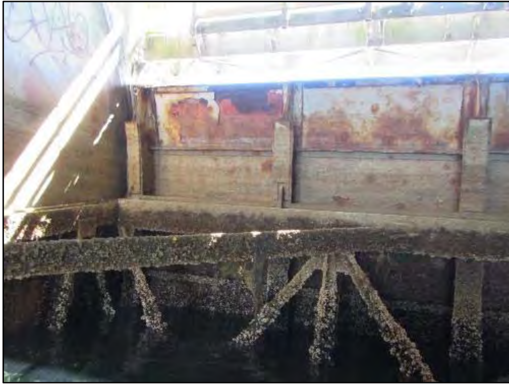
Photograph 19: Inlet Side of West Radial Gate.
