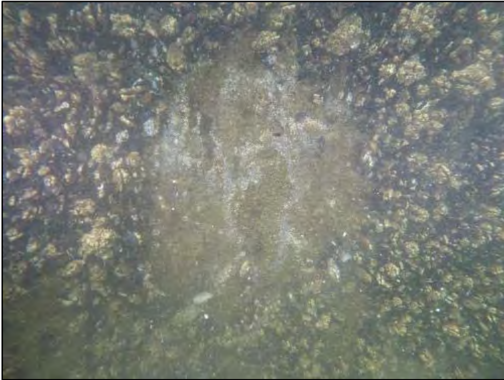
Photograph 44: Level II Cleaning on West Downstream Wingwall
