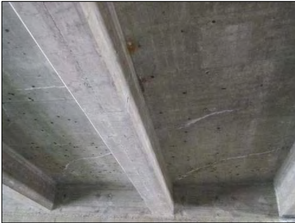
Photograph 15: Typical Girders and Deck Soffit – West Channel
