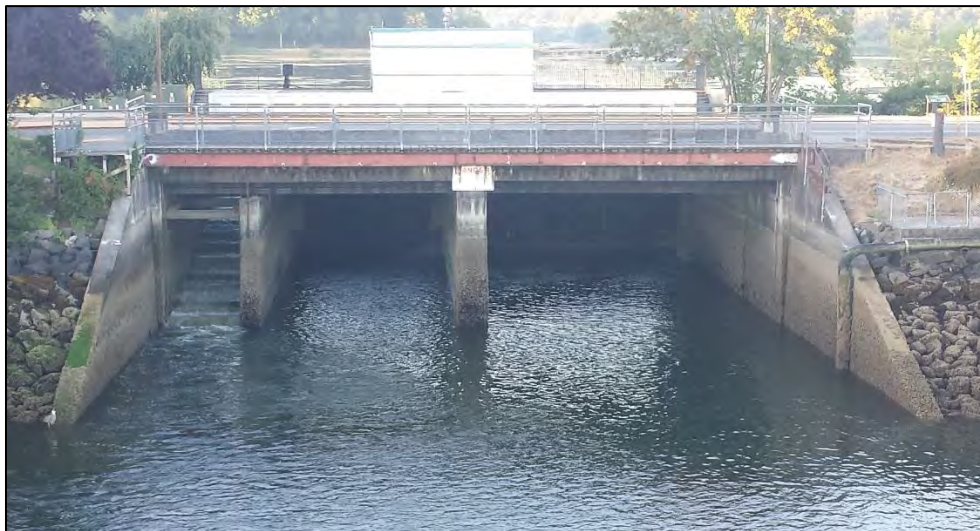
Figure 1: Overview of Dam from the Budd Inlet Side
