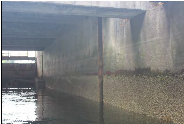
Figure 7: East Channel Pier Wall
