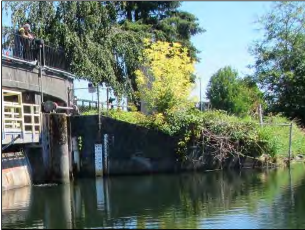
Photograph 40: East Upstream Wingwall
