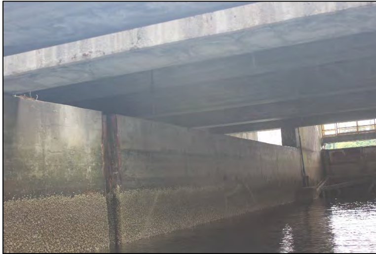
Figure 6: East Channel Fishway Channel Wall
