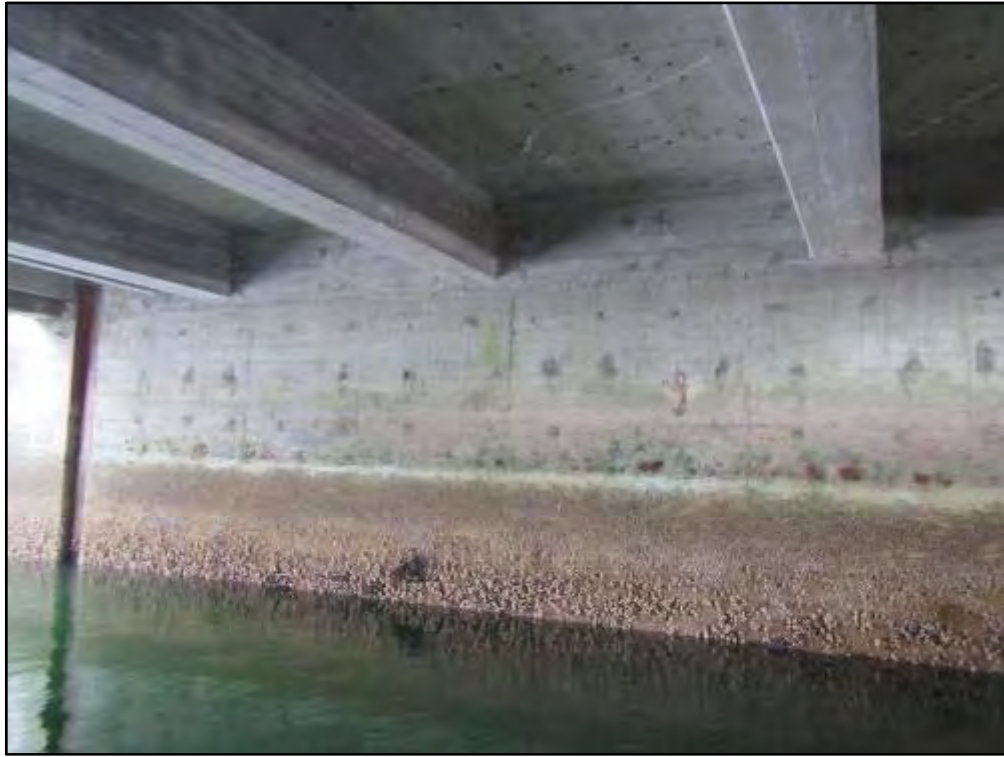
Photograph 2: Typical Pier Wall Looking Northeast
