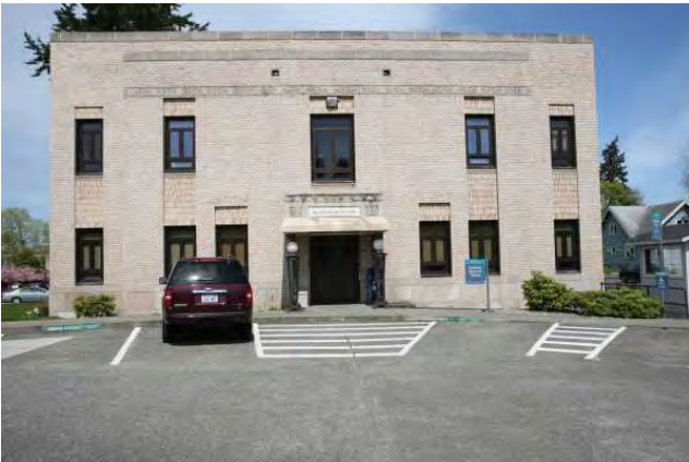
South (rear) facade
