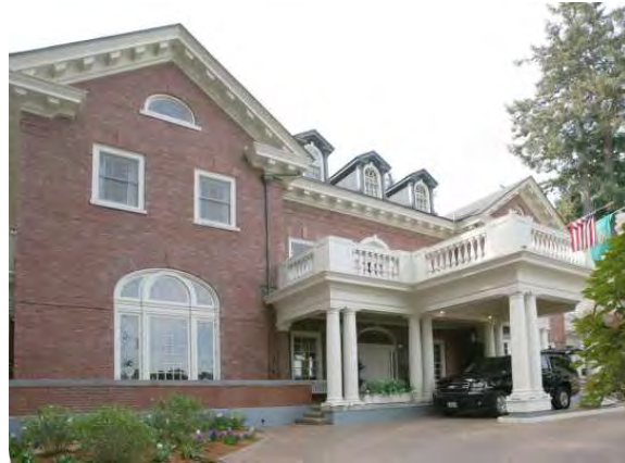
Front (north) facade
