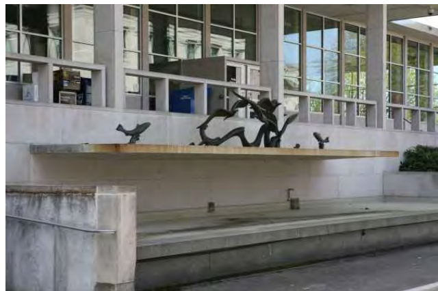
DuPen fountain on the front (north) facade
