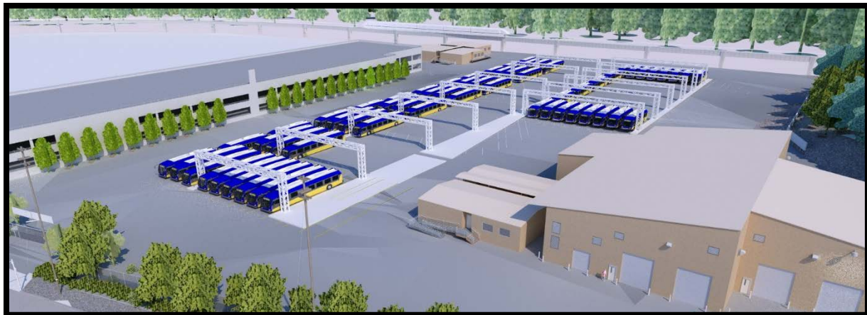
Image 2. Overview of IBE site, looking East, electric buses with gantries.
