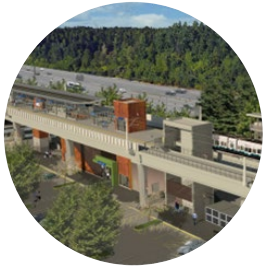
Federal Way Link Extension
