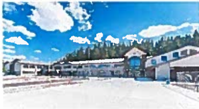
Clover Park School Dist., Hillside Elementary School (GC/CM) JBLM/Lakewood, WA
