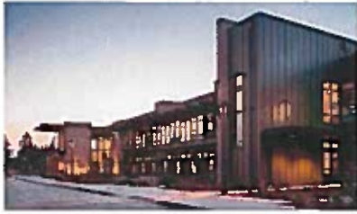
Mason County PUD3, Johns Prairie Operations Center (GC/CM), Shelton, WA
