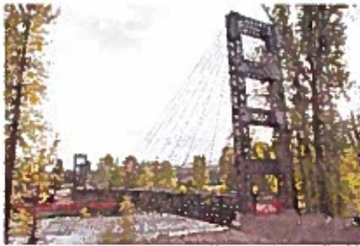
Spring Creek Pedestrian Bridge (Design-Build) Winthrop, WA
