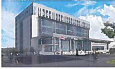
Snohomish County Courthouse (GC/CM) Everett, WA
