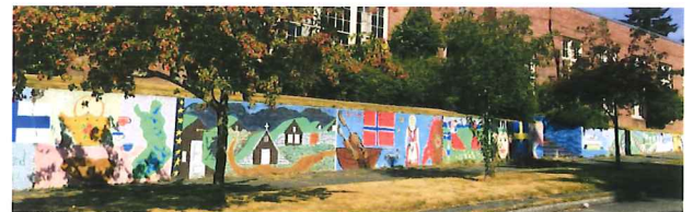
Retaining wall on East side
