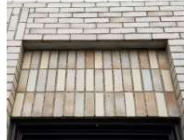
Variegated glazed bricks from façade.
