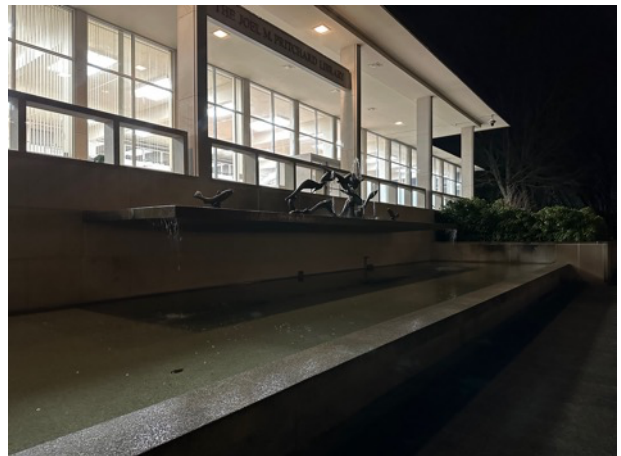
Fountain at night with no lighting operative.
