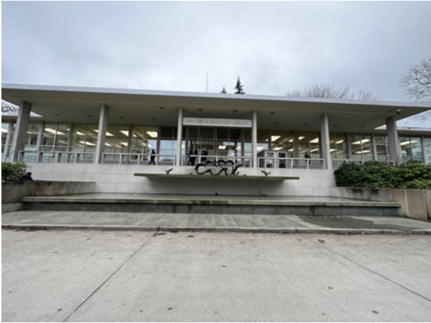
Overall of the whole fountain from the front.
