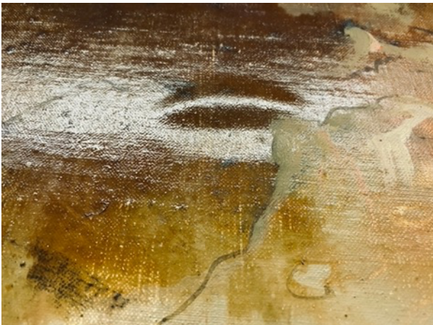
Detail of area where the adhesive seems to have migrated through the canvas to the surface (brown discoloration) as well as an air pocket between the canvas and wall.
