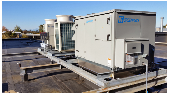
Mechanical Upgrades & Replacements, South Seattle College
