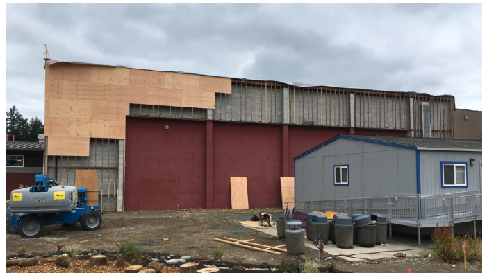
Envelope Improvements, Capital High School, Olympia School District
