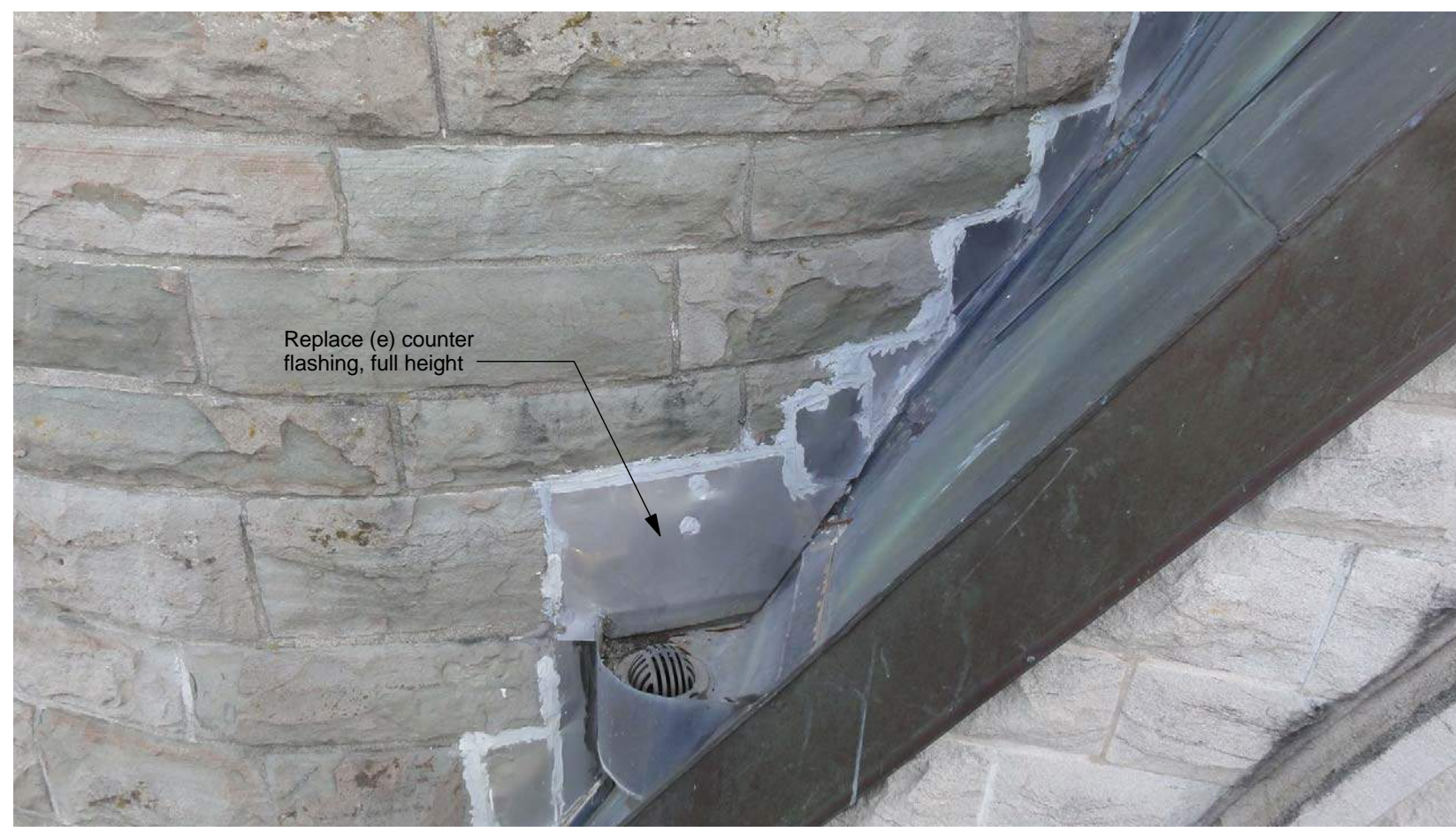
14 West Tower Drain Existing Conditions Alternate No.2
