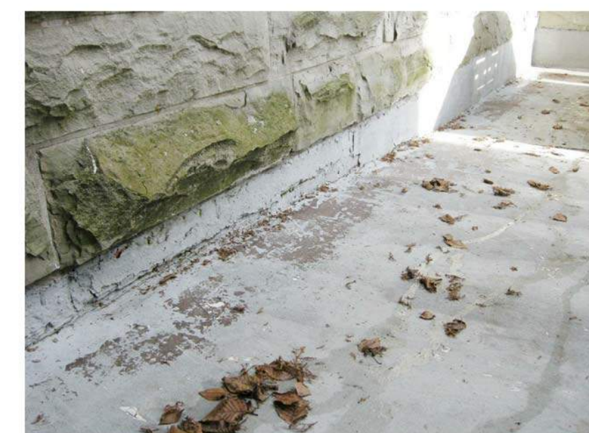
11 (e) North Section of Mech. Room Existing Conditions
