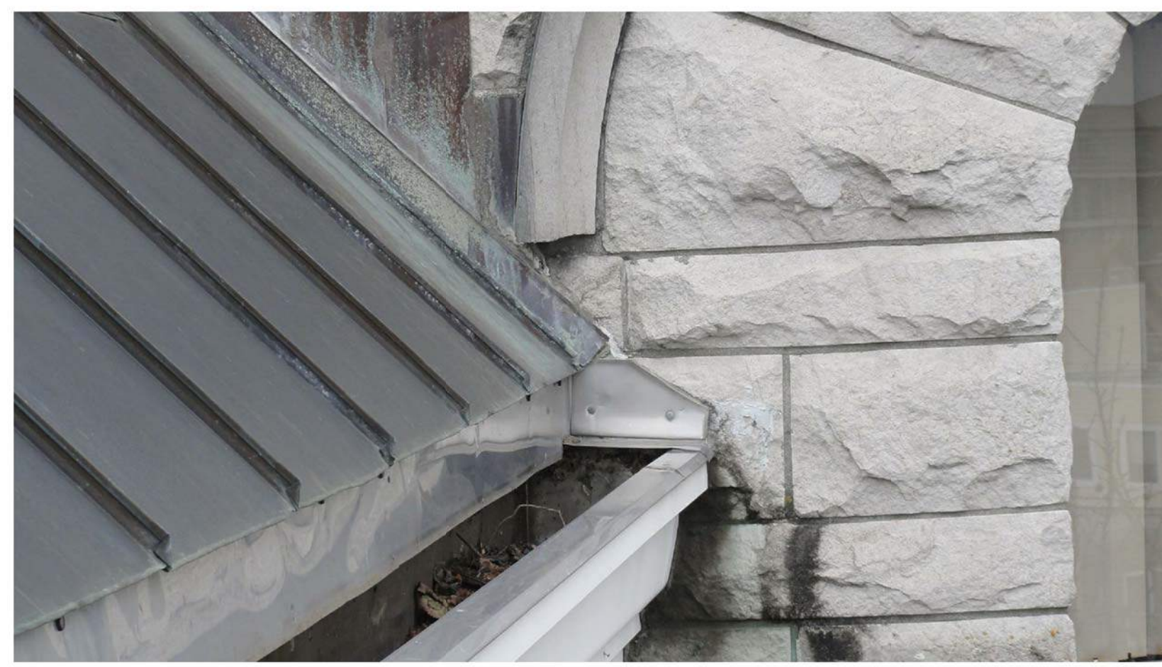
10 East Tower Gutter Existing Conditions
