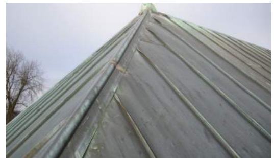
Figure 6. Ridge cap transition with sealant
