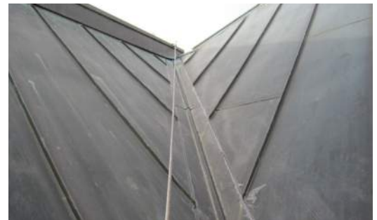
Figure 4. Valley flashing
