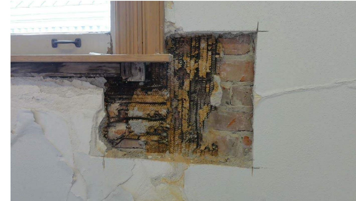
1 (e) Condition - Cut Plaster at Stairwell
