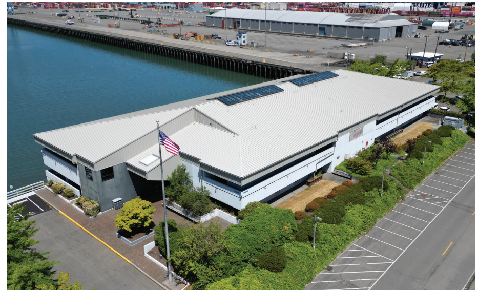
New standing seam metal roof
