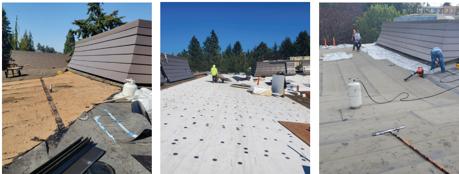
Sequence photos of the 5000 Building Membrane Re-roof
