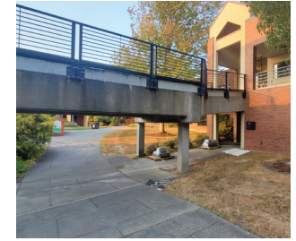
Repaired Pedestrian Bridge
