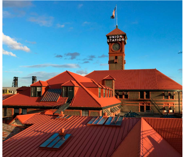
View of Portland Union Station from the north. All skylights were replaced with new skylights to match historic. Lacey Glass provided the custom skylights.
