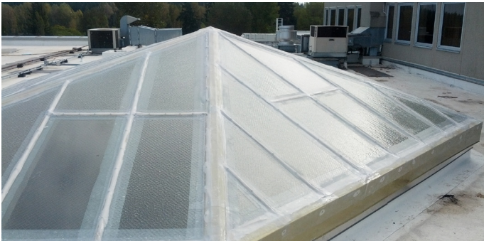
Skylight Replacements, Pierce College
