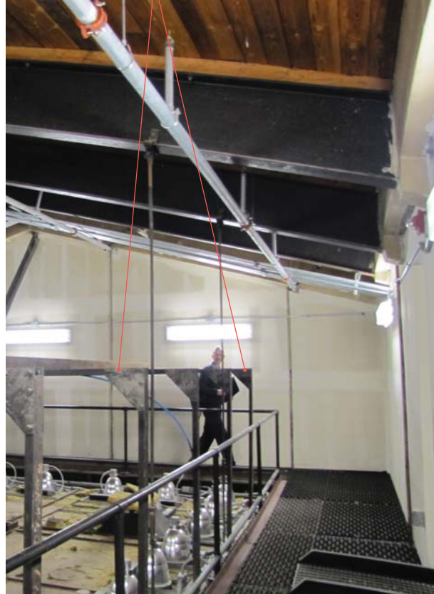
Figure 28: Catwalk and pipe rail around ceiling laylight
