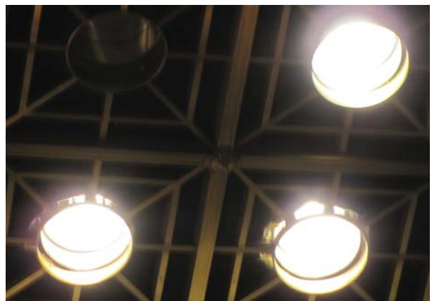
Figure 21: Light leaks / misalignment of downlights
