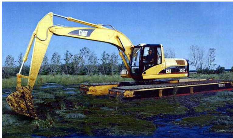
Figure 10. Excavator dredge on track-mounted barge
