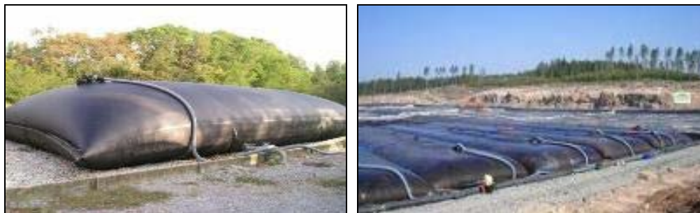
Figure 17. Geotubes used in dewatering (source: Tencate)
