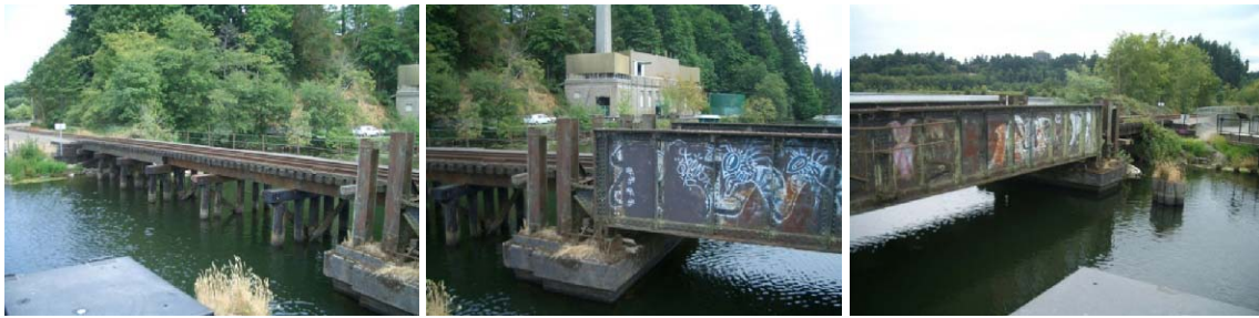
Figure 13. BNSF Railroad Trestle
