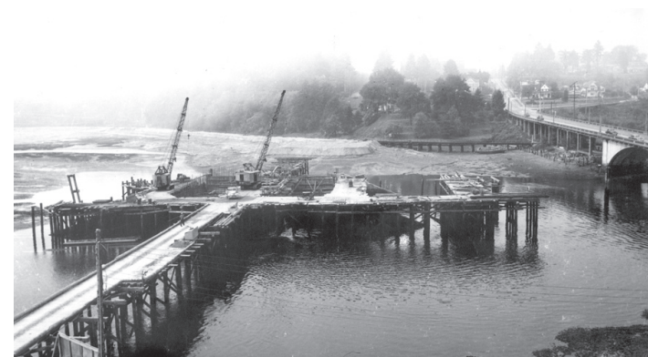
Construction of the Capitol Lake Dam, 1950-51. Courtesy of the Washington State Archives, Susan Parish Collection.
