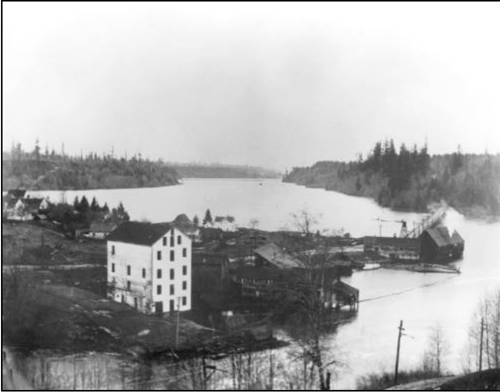
Photo 2-8. Old Crosby Mill in Tumwater looking north with wooden bridge to Old Oregon Trail Road. c. 1909. Courtesy of the Washington State Capital Museum.
