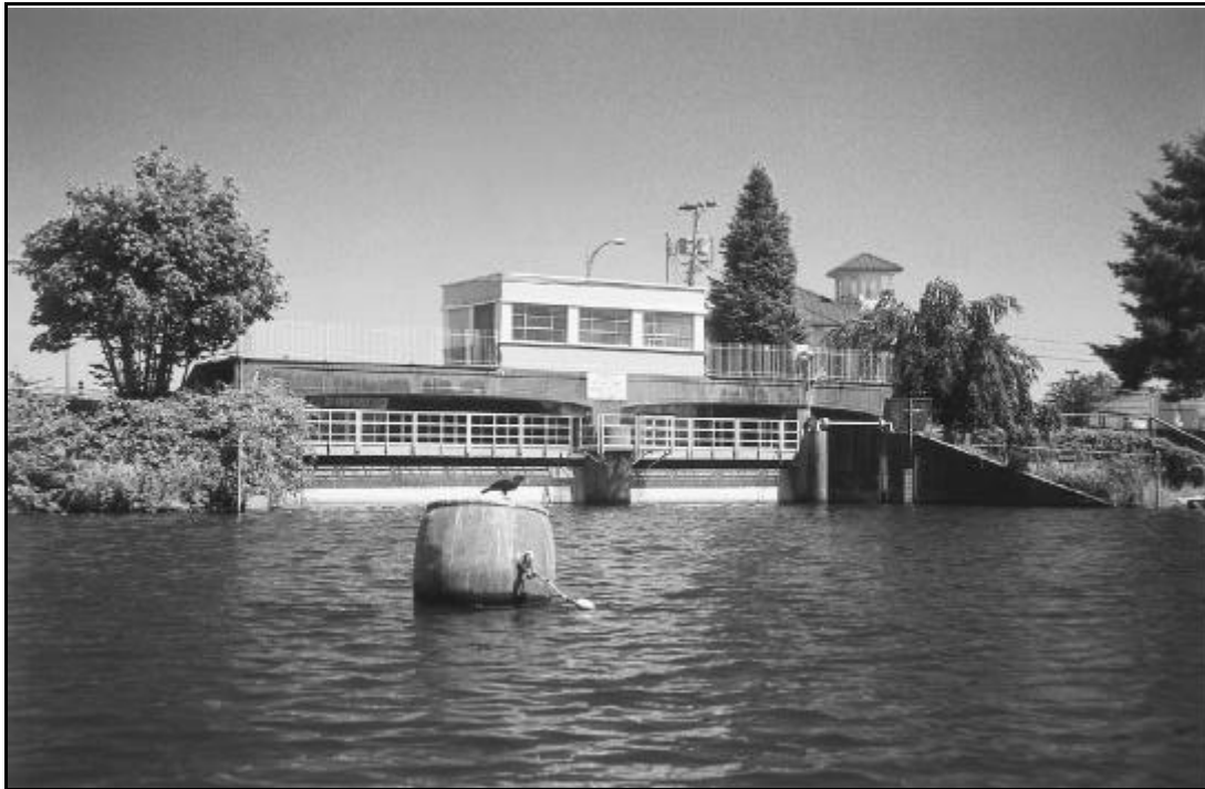
Photo 5-2. Capitol Lake dam from the lake side. c. 1998. Courtesy of General Administration.
