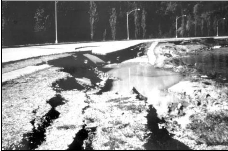
Photo 3-4. Earthquake damage to Deschutes Parkway. c. 1965. Courtesy of Washington Department of Natural Resources.
