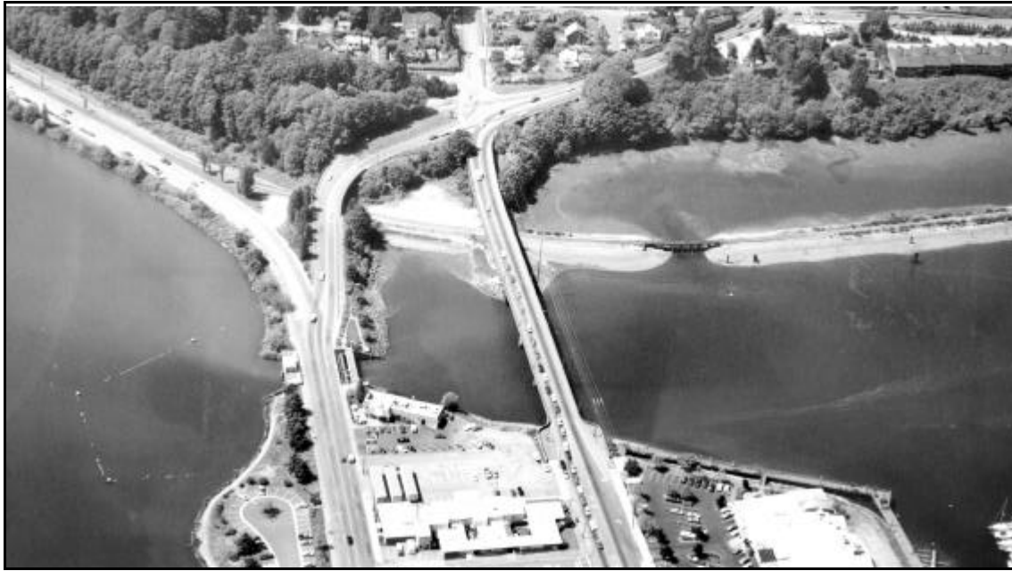
Photo 3-9. Aerial view of the 4 th and 5 th Avenue Corridor and Capitol Lake Dam. c. 1992. Courtesy of the Washington Department of Ecology.
