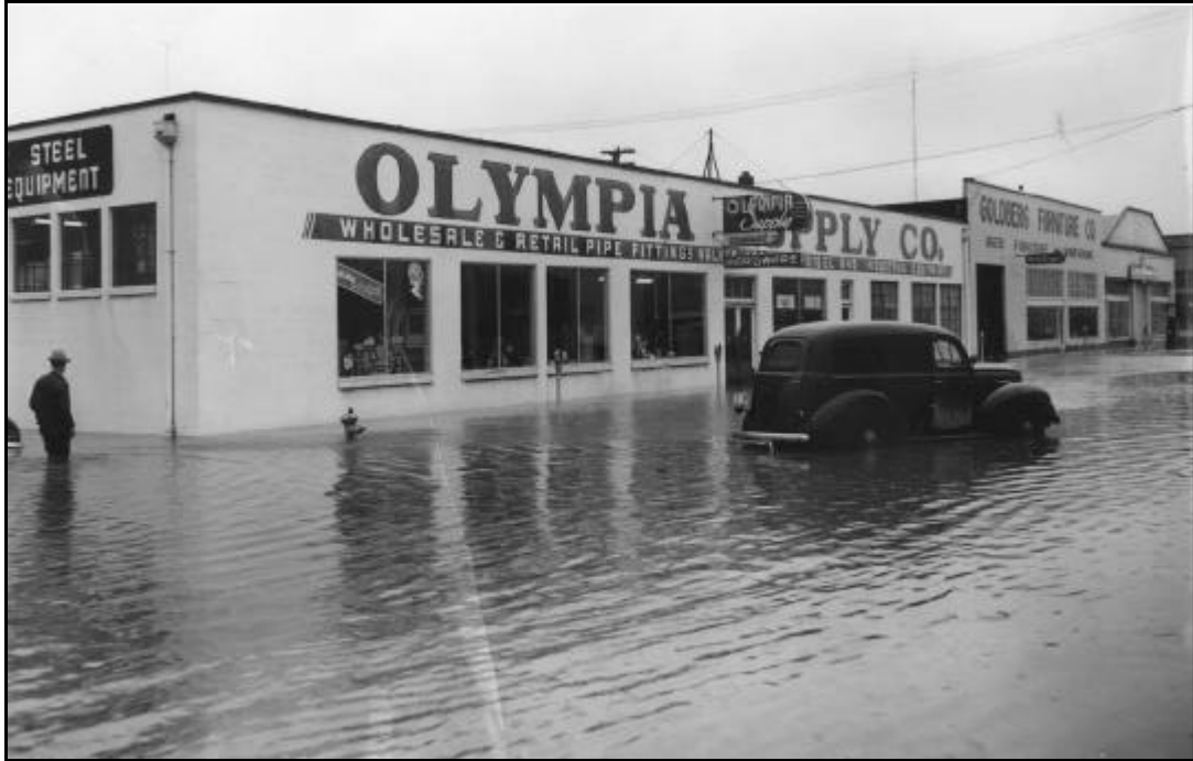
Photo 5-3. Flooding at corner of 7 th Avenue and Columbia Street (June 1951). Courtesy of Susan Parish Collection.
