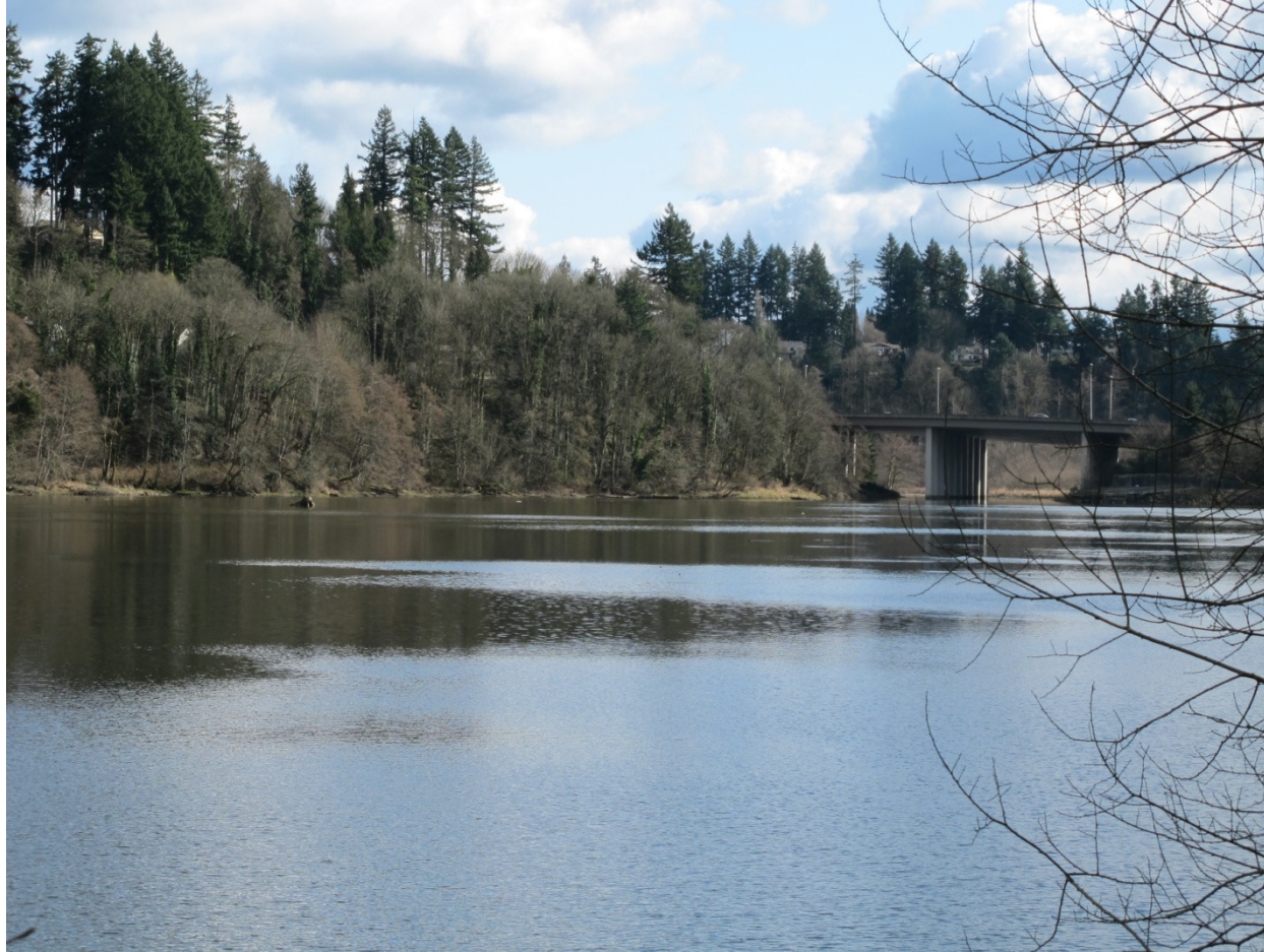
Photograph 1. The Interstate 5 bridge, seen here from the Middle Basin, crosses the narrow channel between the Middle and South Basins.
