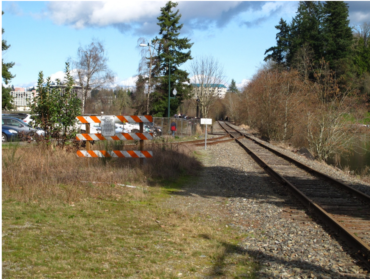
Photograph 8. This area, just south of Marathon Park, on the railroad right-of-way would allow mobilization into the Middle Basin for a heavy lift crane to launch dredge equipment. If sediments had to be offloaded from the Middle Basin for upland disposal or reuse, they could be craned ashore here, treated as necessary, and loaded from Marathon Park (refer to Section 3.4.5 for Off-site Reuse or Disposal Considerations).
