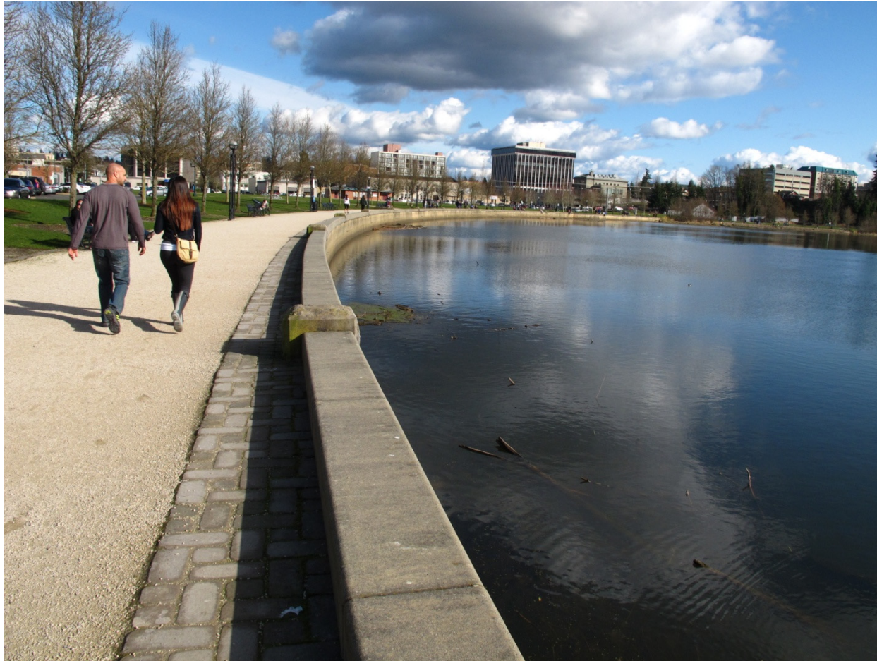
Photograph 6. The walking path and ornamental bulkhead around the North Basin from the dam around to downtown Olympia and Heritage Park could provide access to the North Basin from public streets, but the entire area is a well-developed and heavily-used urban park.
