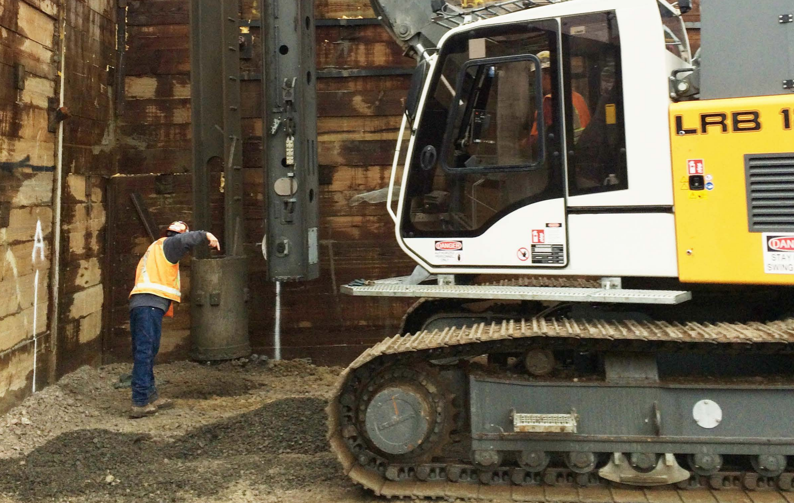
Crews at the 1063 Capitol Way project began drilling GeoWells in November 2016.
