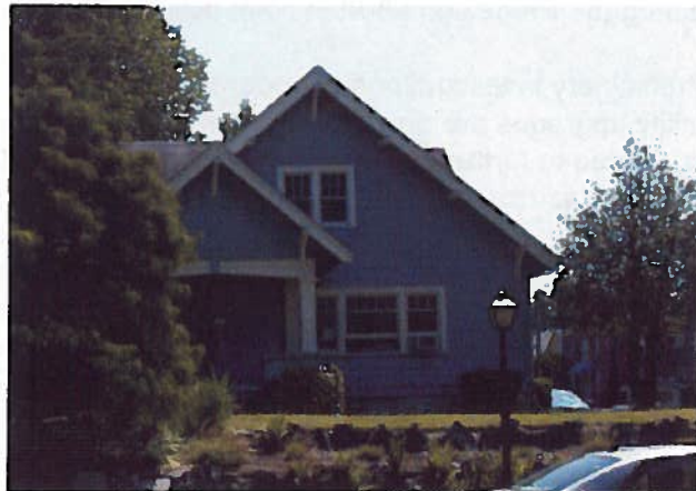
Figure #13 201 14th Ave. - the Blue House, North Facade
