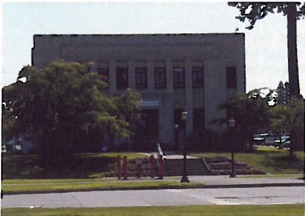
Figure #12 Irv Newhouse Building, North Facade
