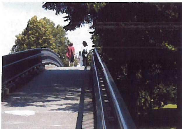
Figure #15 Existing Capitol Way Pedestrian Bridge
