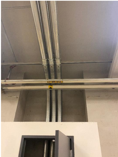
Image 1 – Conduits from LSC Comm Room to Pull Box
