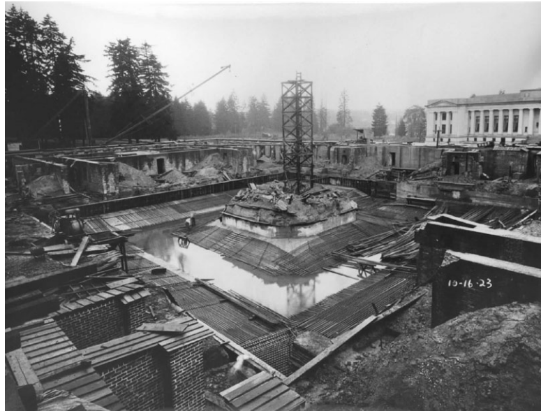
Photo 2- Installation of new Capitol Building foundation, 1923. On file at: https://www.sos.wa.gov/legacy/legbuilding/construction.aspx
