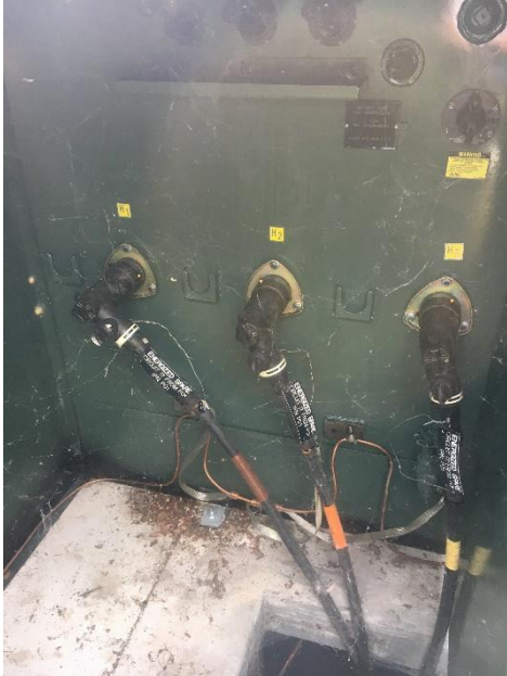
Figure 1 – Vault PN Medium Voltage Transformer
