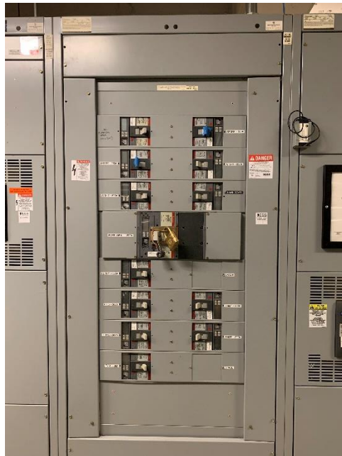
Figure 3 - West Electrical Room MPDH
