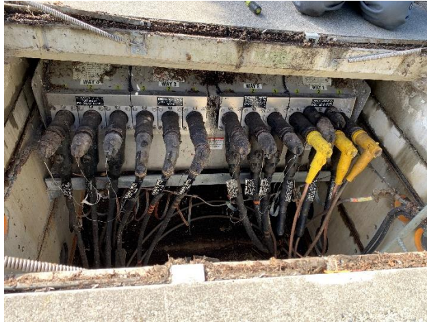
Figure 2 - Vault POX MV Switch
