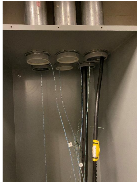
Image 2 – Interior of Pull Box
