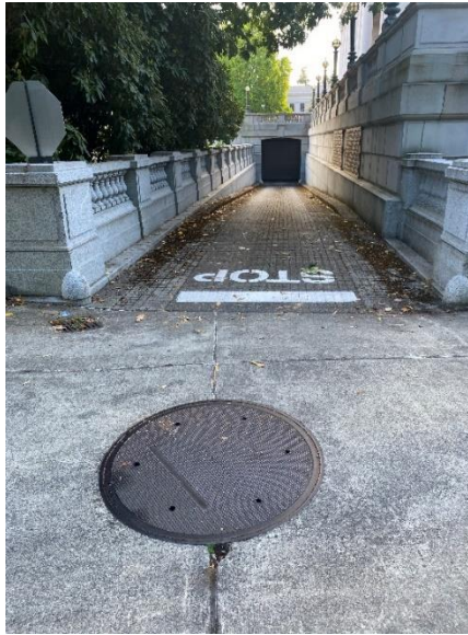
Image 3 – Manhole B Location
