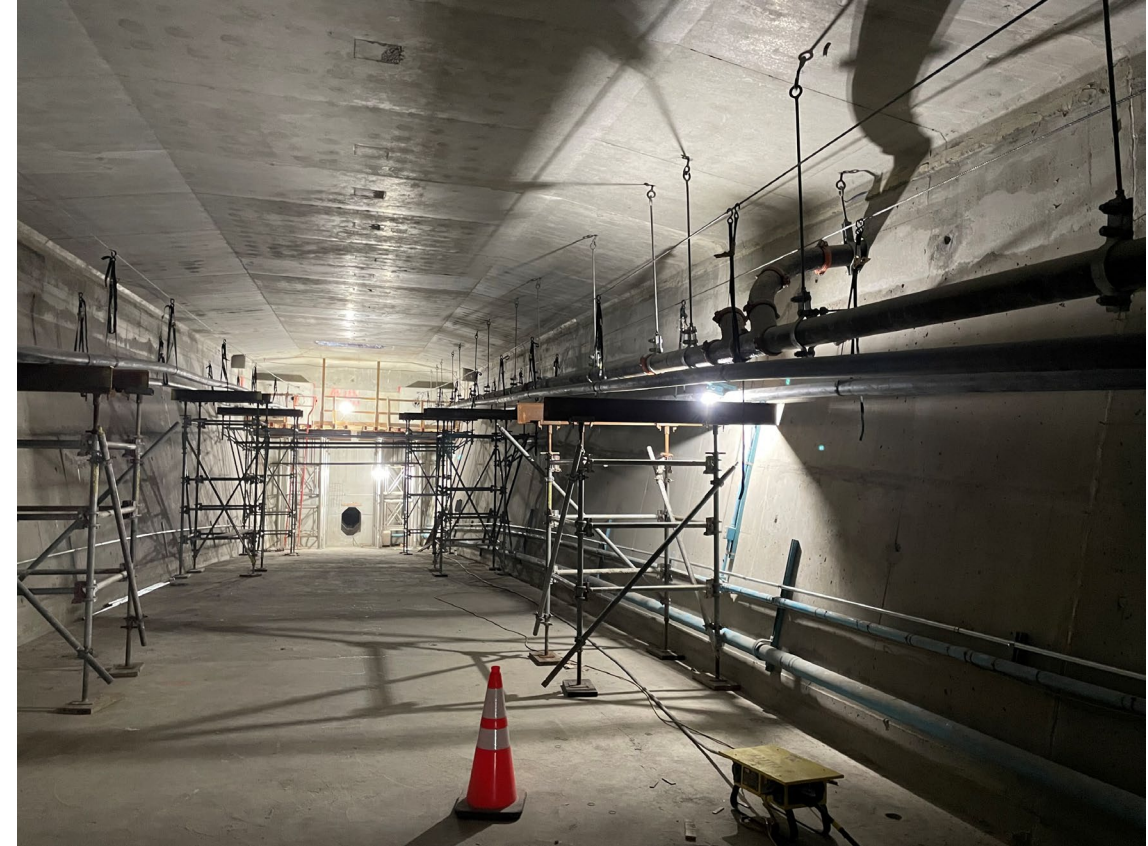
Above: Interior view of the West Seattle Bridge structure
