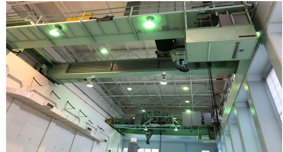
Existing Gorge Powerhouse Crane
