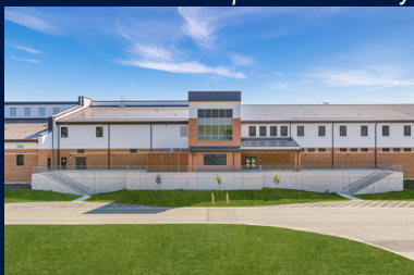
FY20 SOF 22 STS Operations Facility
