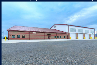
Tactical Equip. Maintenance Facility
