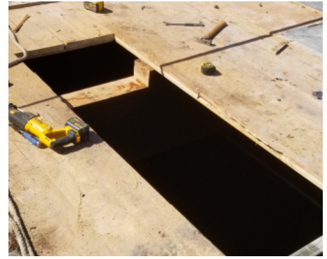
Structural rot repair, Cascade Building Roofing Replacement emergency project - Criminal Justice Training Commission (2019-21 DES On-Call)
