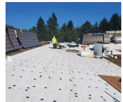
Top Left: Station Bay with rendering of proposed location for the new units; Top Right: Existing Station bay with a fire truck showing the tight clearances; Bottom Left: Aerial of the Re-roof; Bottom Right: Roof board and base ply application
