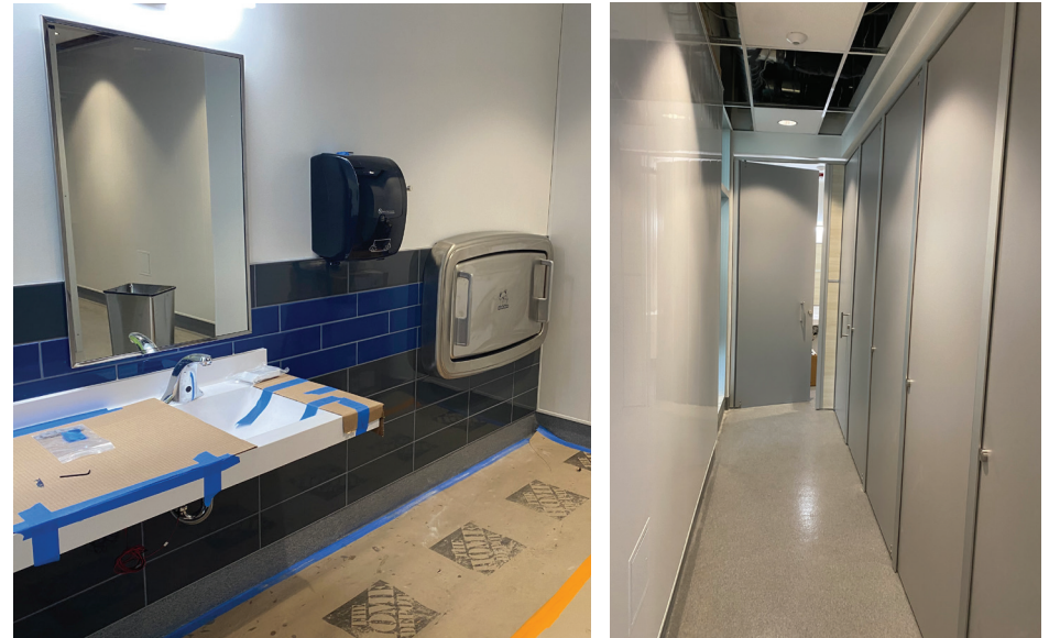
Left: "Trough" sink during construction; Right: New full height toilet partitions
