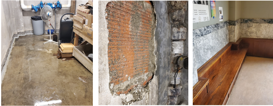
Left: Flooded storage room; Middle: Deteriorated cast iron roof drain embedded behind a layer of clay tile within a historic interior wall; Right: Historic elements prevented replacing or rerouting.
