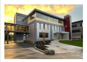
Key updates included the addition of a new entry and a standalone, seismically separated elevator structure. This design not only creates a more prominent focal point for the building but also enhances accessibility for students across all floors.
