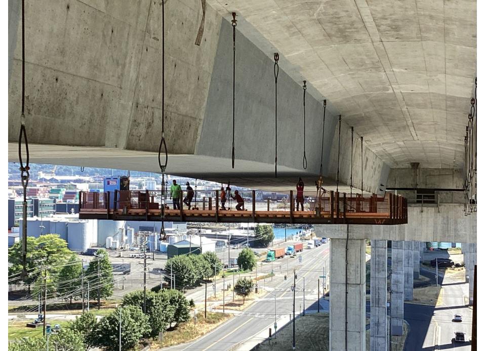
Above: the mobile work platform for under deck work on the West Seattle Bridge GC/CM project.
