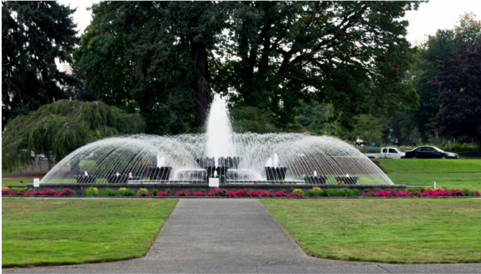
Tivoli Fountain Renovation | Design through Construction - Site Workshop Completed September 2017
