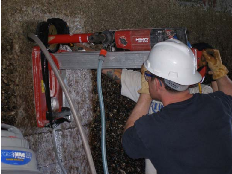
Figure 3. Over-Water Core Drilling
