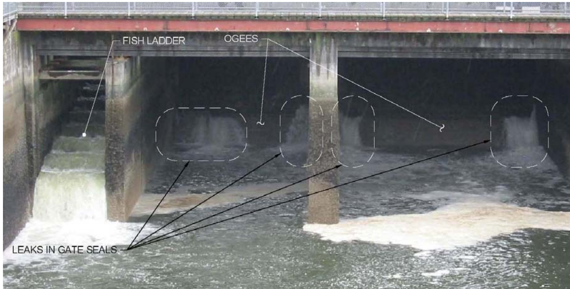
Figure 9. Radial Gates As Seen From Budd Inlet Side During Low Tide
