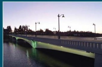
Removal of the 5th Avenue dam will require new bridge construction, south of the 4th Avenue bridge erected after the 2001 Nisqually Earthquake Photo: City of Olympia
