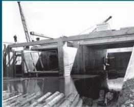
5th Avenue Dam under construction in 1951 Photo: Thurston Regional Planning Council
