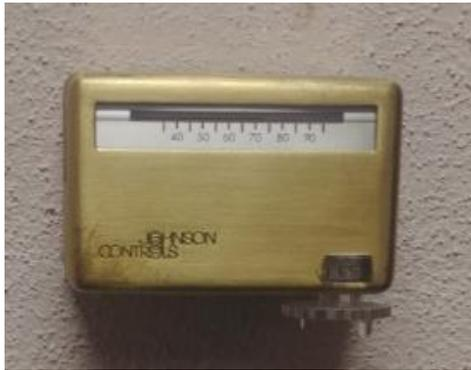
*Pneumatic Thermostat (Installed in 1987)*
