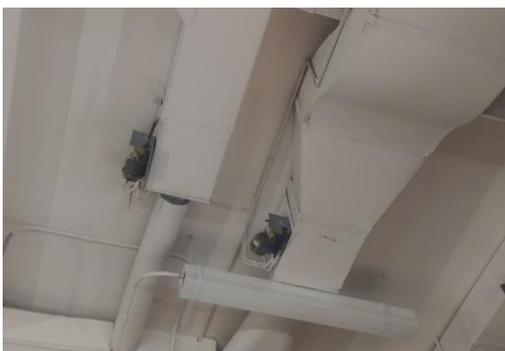
*VAV Boxes (box with a pneumatic damper)*
