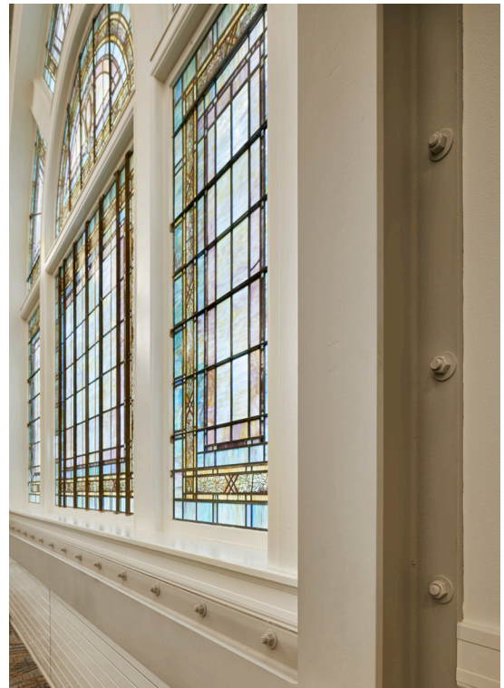
□ Town Hall Seattle's historic preservation included the rehabilitation of monumental stained-glass windows in the Great Hall. Out of plane bracing was carefully shaped to frame, rather than block, the arched of the windows.
