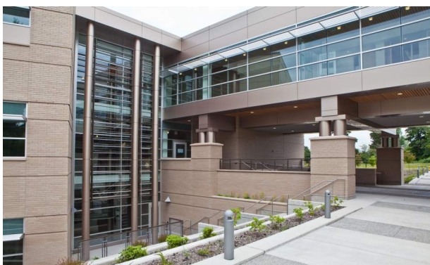
Top to bottom: SVC Laura Angst Hall Chemistry lab; CWU Samuelson informal learning spaces; LWTech Allied Health Building accessible pathways on each of three levels
