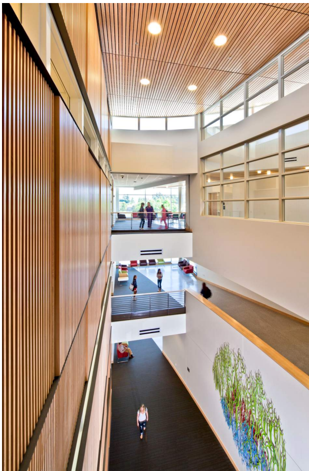
Allied Health Building, LWTech
