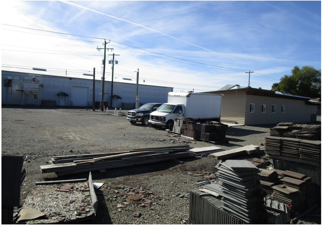
Building 603, Building 605 and Yard Ahead
