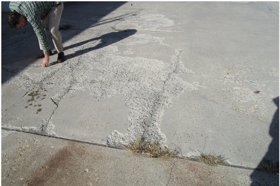
Concrete Paving On Site
