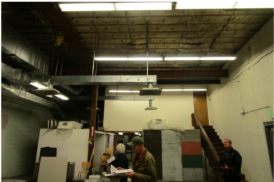
Building 602 - Lab Space
