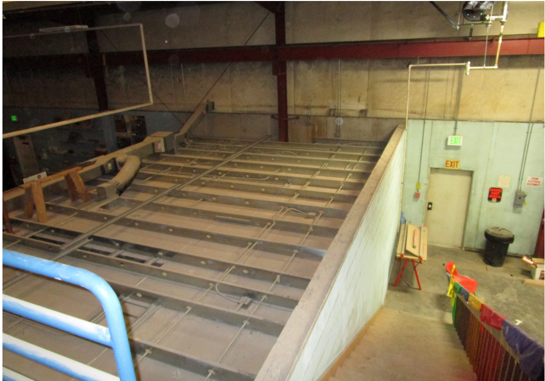
Building 603 - Typical Stair
