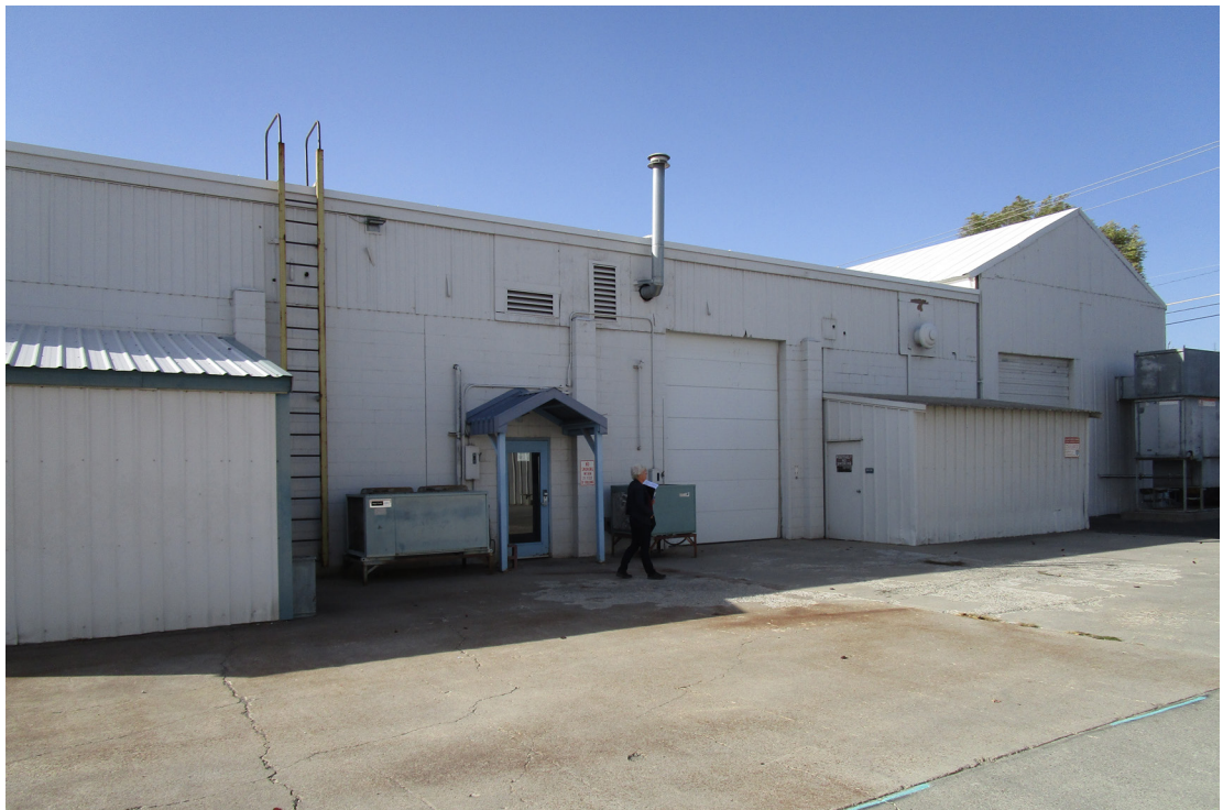
Building 602 and Metal Building Addition
