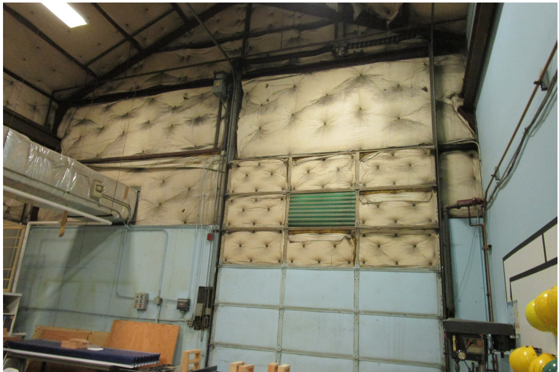
Metal Building Addition to Building 602 - Lab Space
