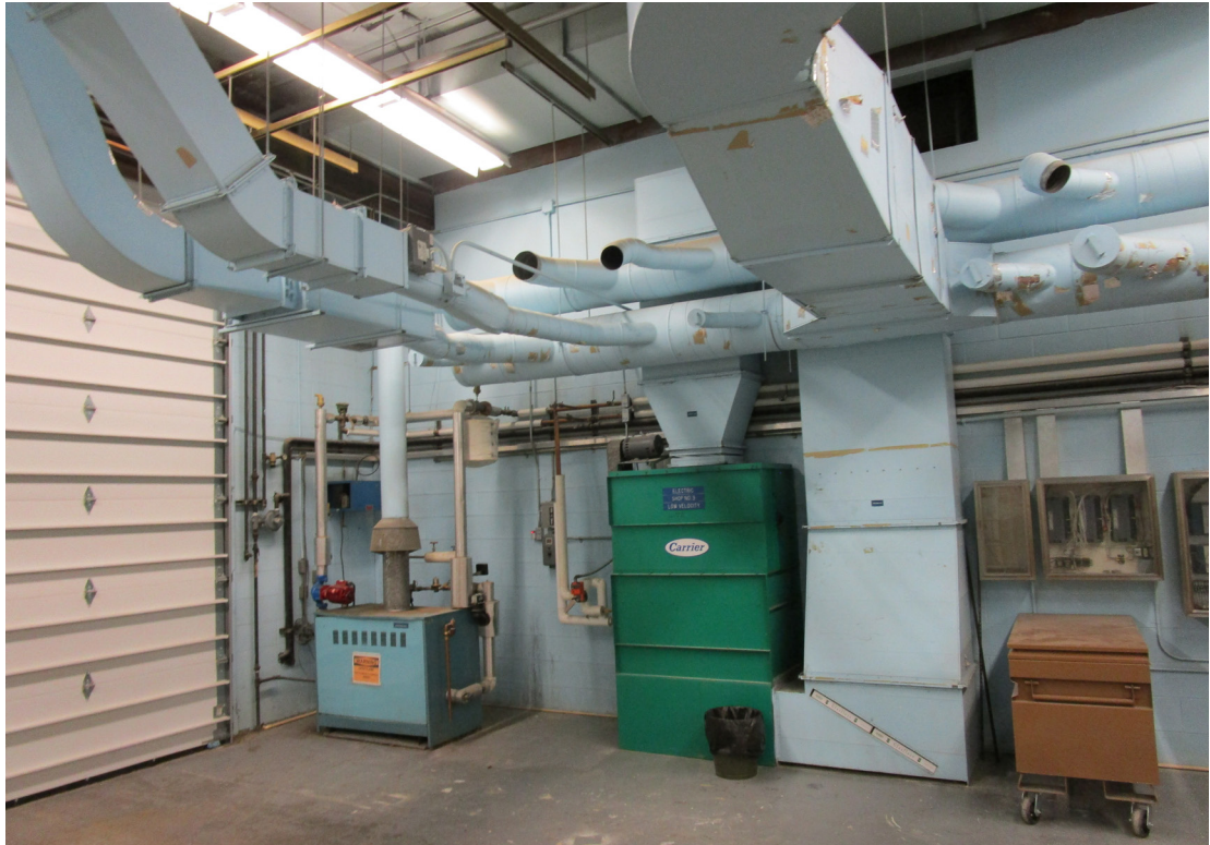
Building 602 - Mechanical Equipment
