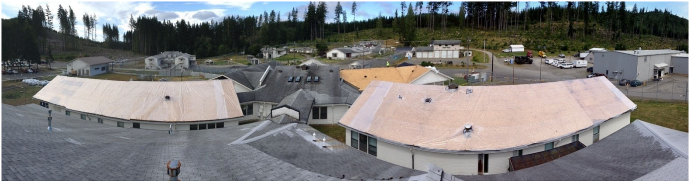
Cedar Creek Corrections Facility – Cascade Building Re-Roof
