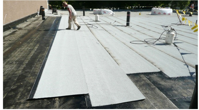
Centralia College Gymnasium Re-roof -Built up -Roof Centralia, WA
