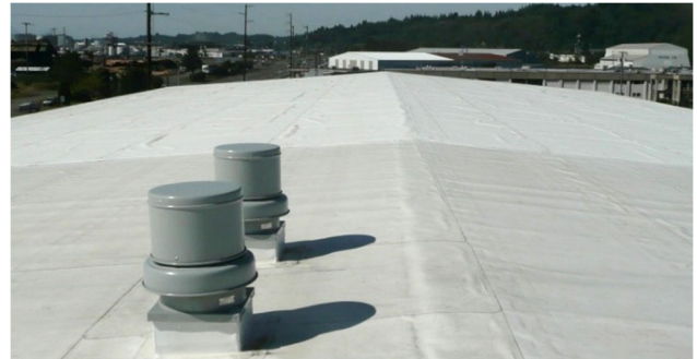
Port of Grays Harbor R&D Facility Single Ply Re-Roof Aberdeen, WA
