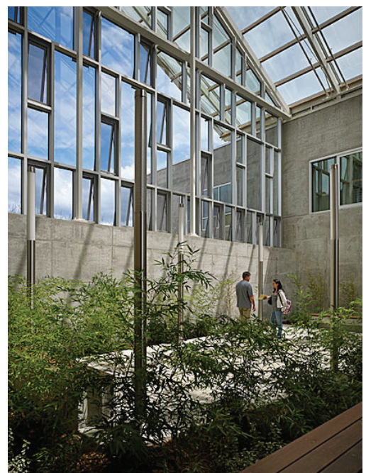
Winter Garden natural ventilation space Rainier Science and Technology Building Pierce College, Ft. Steilacoom
