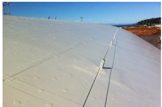
Port of Olympia Terminal A Warehouse Single Ply Re-Roof Olympia, WA
