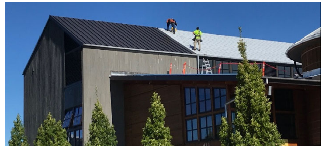
Hands-On Children's Museum Re-Roof Olympia, WA
