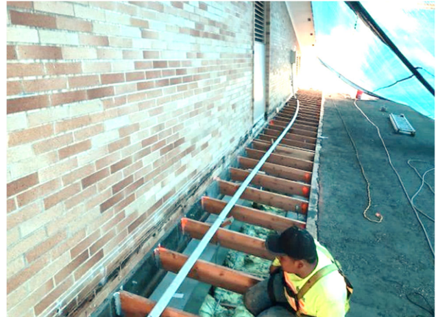
A worker installs epoxy-set anchor bolts strengthening the connection between the roof and masonry wall LDS Church Issaquah, WA
