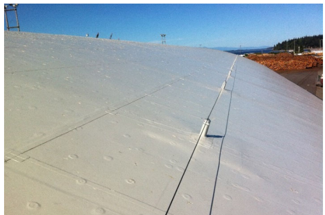
Fall Protection, Marine Terminal A Warehouse
